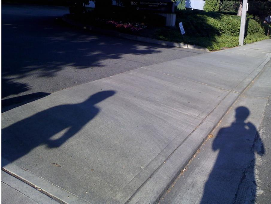
Bellevue Curbs: Curb outside BCC on Northrup Way (next to Burger Master). The ramp has about a two inch or so lip instead of being flush with the street. This makes it hard for bicycles (especially road bikes) to go up the ramp from the street. It in fact led to a nasty road rash on my arm. The bicycle must enter the ramp at a large enough angle for the tire to hop-up the extra few inches. [nyhokie]
