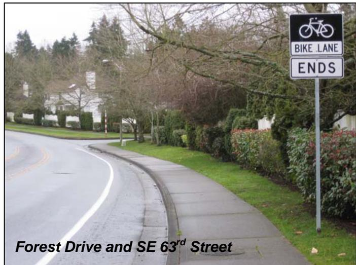
Between SE 63<sup>rd</sup> Street and 152<sup>nd</sup> Avenue SE Forest Drive consists of two travel lanes that occupy the 34 foot wide roadway for most of the corridor (several instances of center turn lanes). This corridor is envisioned as having bicycle lanes reflected in the new Pedestrian and Bicycle Plan which proposes project **B-158-N/S** which would add a 5 foot wide bike lane on the north side of Forest Drive SE from SE 63<sup>rd</sup> Street to Lakemont Boulevard SE..
