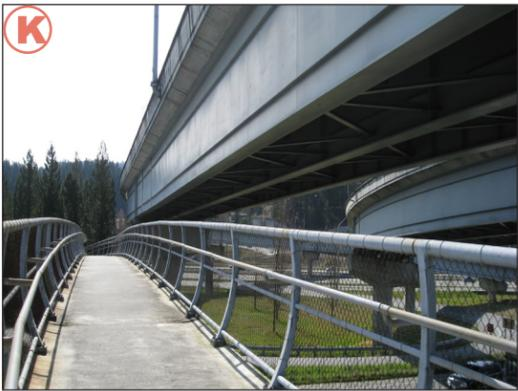
The on and off ramp infrastructure built at the 148th Avenue SE, SE Eastgate Way and I90 area includes an overpass solely for pedestrians and bicyclists.
