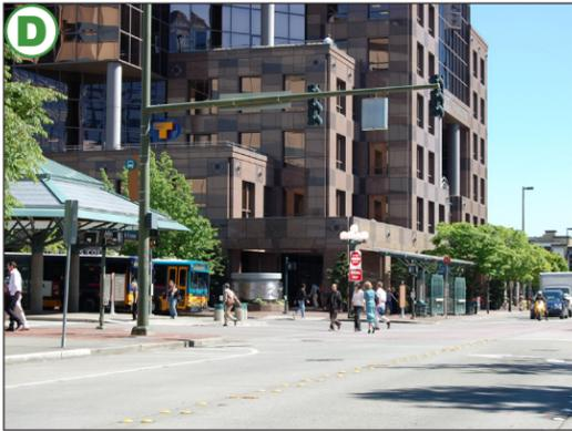
Perpendicular to NE 6th Street, 108th Avenue NE has a large right-of-way. The travel lanes in both directions are 14 feet wide, in addition to a central turning lane, both of which support the high volume of bus traffic in this area near the transit center. Bicyclists must navigate a scramble crosswalk and bus activity, which can be especially challenging during peak hours. (facing south, pg 30)
