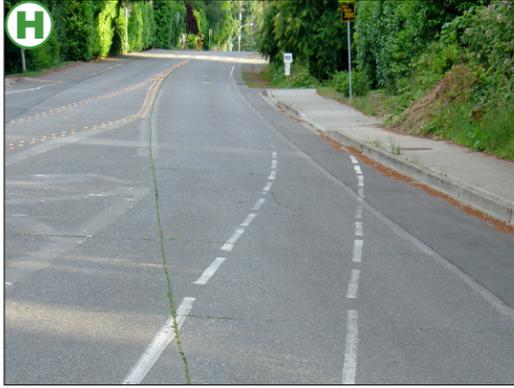
The bike lane at 108th Avenue NE and SE 21st Street completely disappears after the intersection, as does the sidewalk. This forces bicyclists into a dangerous situation of merging into moving traffic without warning. (pg 31)
