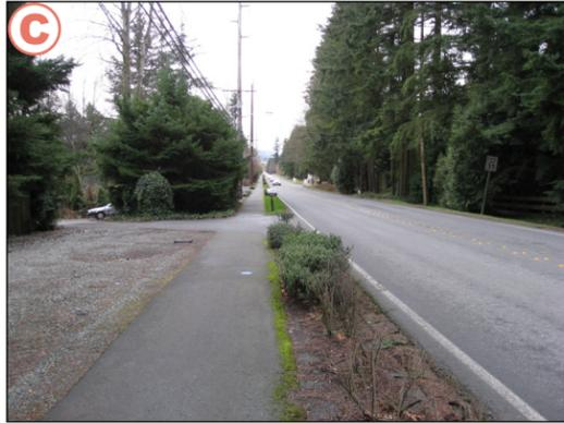
Looking north, the recently constructed 6 foot-wide porous asphalt pathway and planter strip/buffer can be seen on the west side.
