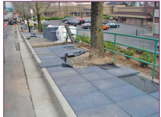
***Rubber sidewalk panels — made of recycled tires — at NE 10th St west of 102nd Ave NE allow tree roots to grow under the sidewalk without creating a trip hazard.***
