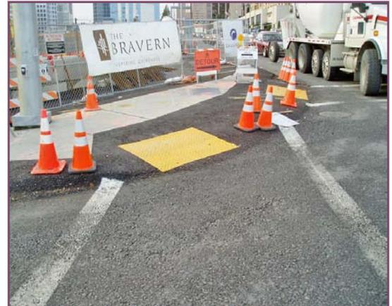
*A temporary curb ramp provides pedestrians with disabilities with a continuous route through a construction area.*
