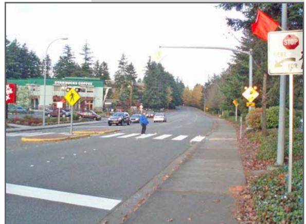
***The placement of the stop bar set back from the crosswalk together with “stop here for pedestrian” signing and the flashing light system is showing improved driver compliance to pedestrians within the crosswalk.
