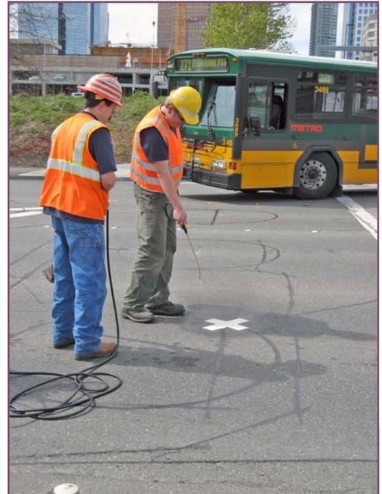
*Bellevue staff applying the torch-down "X" marking the location of a bicycle actuated signal.*
