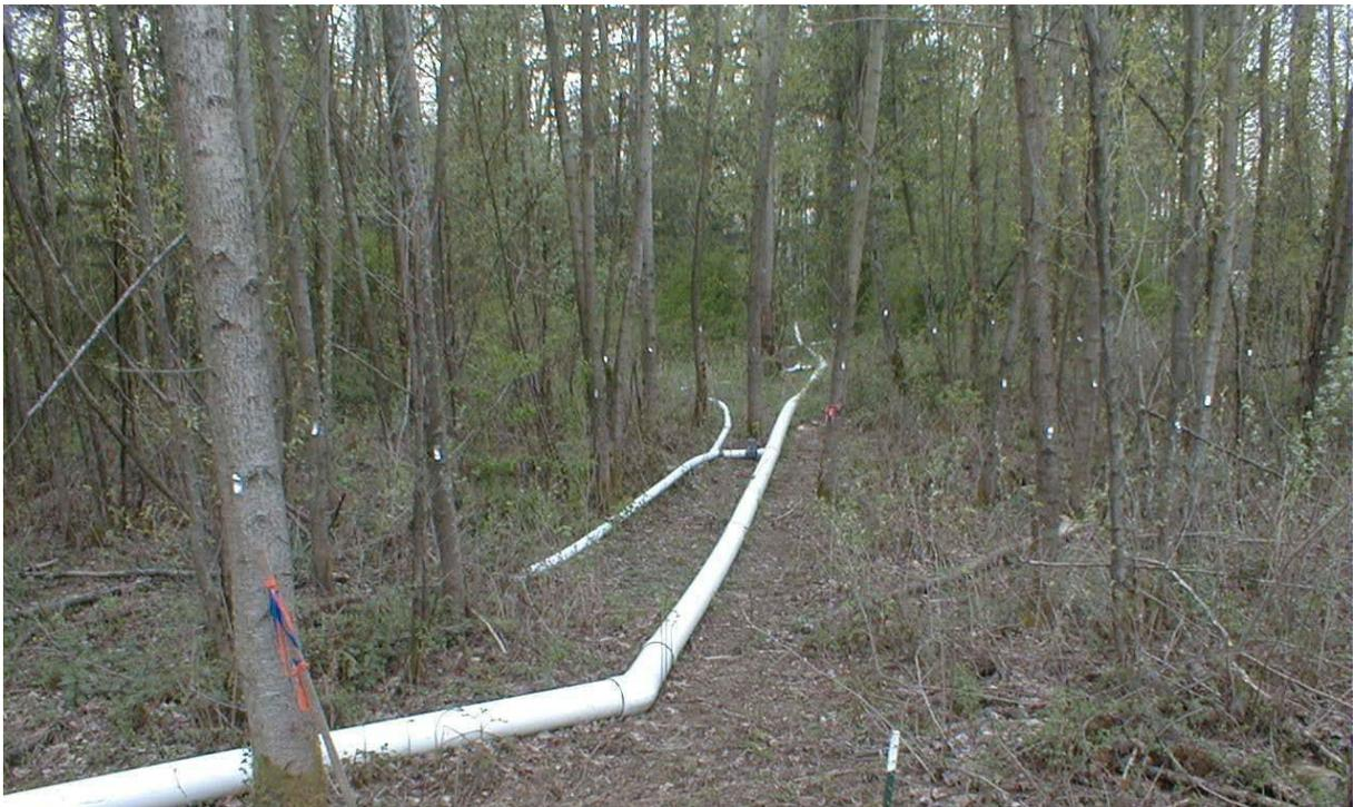
**Figure 4.2.15 – Manifold and Branches in a wooded, vegetated spray field**
