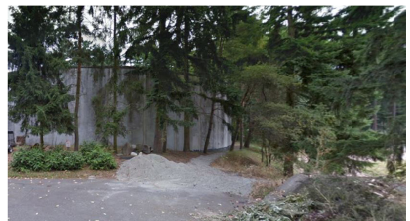
Figure 10.2 - Clyde Hill 390 Reservoir Tank
