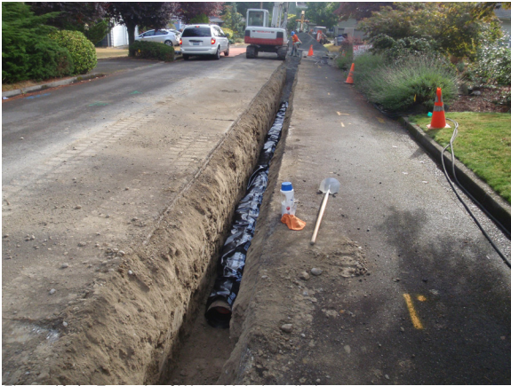
Figure 10.4 - Example of Water Main Installation
