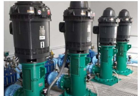
Utilities operates 23 pump stations throughout Bellevue's system. Booster pumps, such as the new ones above, are critical for delivering drinking water, especially at higher elevations in the city, like Eastgate/Cougar Mountain neighborhoods.
