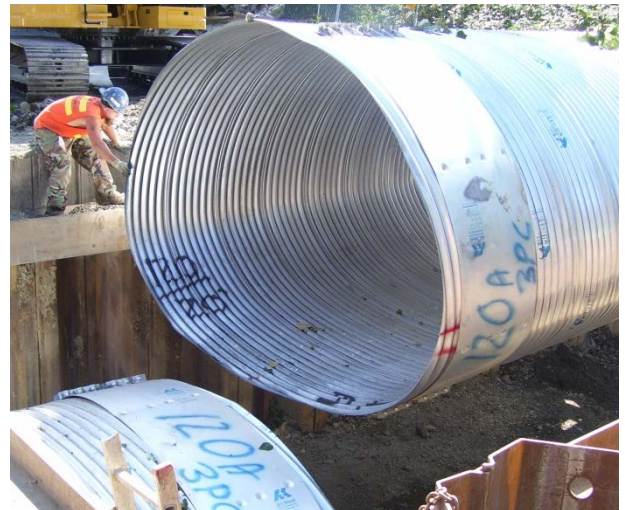
An existing culvert under SE 6 th Street was removed and replaced with a larger culvert to carry Sturtevant Creek and reduce flooding in the area.
