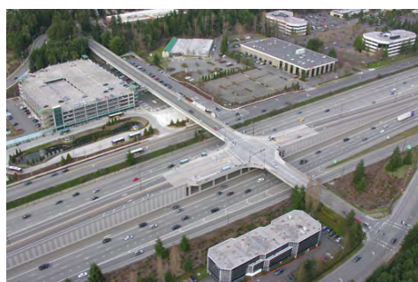
Eastgate Direct Access Ramp (2006) - $19 million
