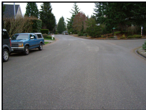
Eastbound on SE 44th PI West of 155th Ave SE
