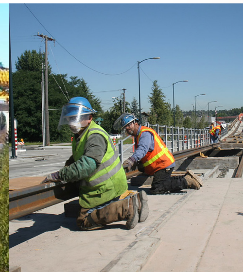
Laying light rail tracks
