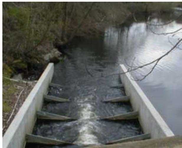
**Figure 2. Mercer Slough fish ladder (site #445) before being reconstructed (photo on left) and after reconstruction (photo on right) in 2003.**
