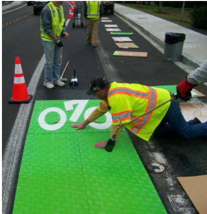
Installation of green bike lanes on SE Newport Way, near 150th Ave. SE.
