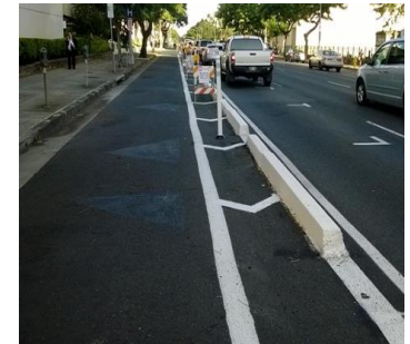
Cast in Place Barrier Curb
