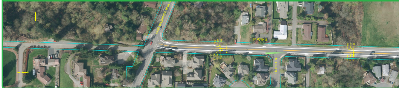
SE 60th St from Lake Washington Blvd SE to 116th Ave SE
