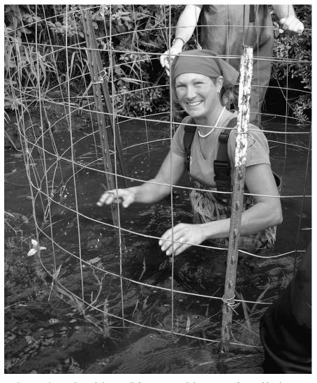
Utilities worker Trish Tyo helps install fencing around the opening of a pond leveler, placed in a beaver dam to allow salmon passage and stream flow.
