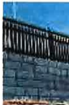
Fabricated Metal Guards on Wall to match Station accessories Guard with galvanized railing positioned on top of low wall to prevent and buffer pedestrians from parking lot adjacent to trail.
