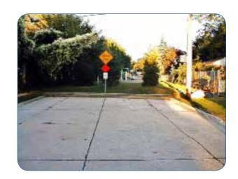
A full closure can be designed to accommodate nonmotorized travel such as pedestrians and bicyclists, as well as access for emergency response vehicles.
