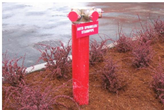
As a general rule, fire protection equipment including fire department connections are identified by a red post and red sign with white letters. The sign shall include the following information:
