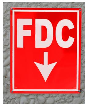
The location of the FDC's may not always be visible from the street or nearest point of fire apparatus access. In those instances, the location of the connection must be clearly identified with approved signage. The letters "FDC" must
