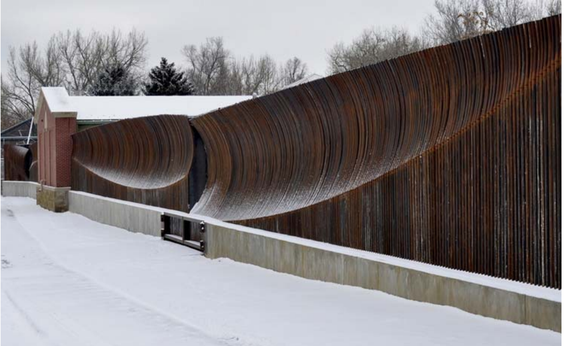
130 th STREET STATION— PLATFORM BAULUSTRADE: PATRICK MAROLD
