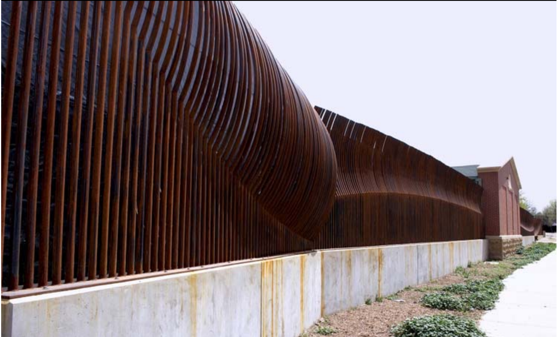
130 th STREET STATION— PLATFORM BAULUSTRADE: PATRICK MAROLD
