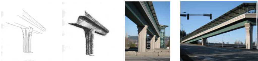
Sound Transit Canyon Park Station implementing I 405 Context Sensitive Design. Construction documents by WSDOT Bridge Office.
