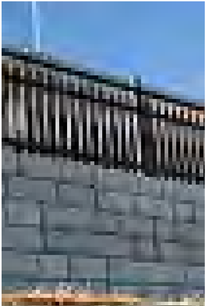
Fabricated Metal Guards on Wall to match Statiion accessories
