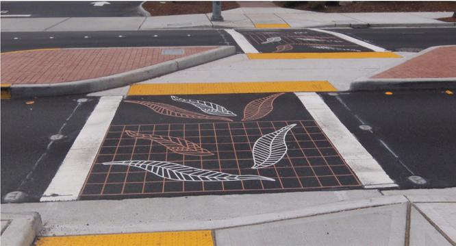
To distinguish the crosswalk from the travel lane and to provide a more interesting and pleasant environment for the pedestrian, special paving is installed in the crosswalk. For added safety the special paving is bracketed by wide and highly visible white lines. The longevity of the pavement design is extended by embedding the decorative pattern into the asphalt so that it is not worn off by vehicle tires.
