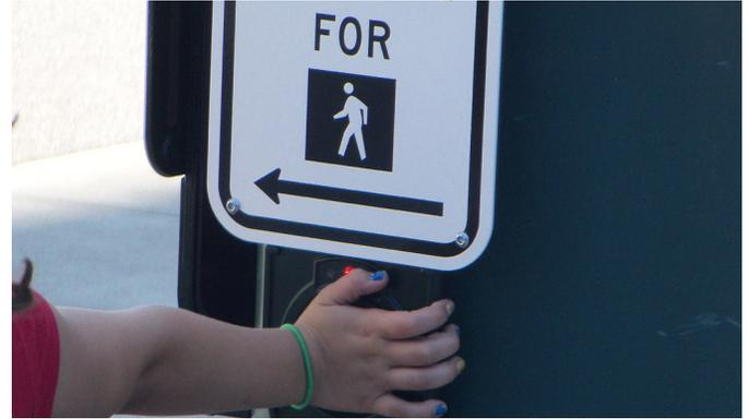
through a green interval if sufficient green time is available in that cycle to allow a pedestrian to cross. The permitted left turn signal phase for vehicles is skipped when a pedestrian is served as an additional safety measure.
