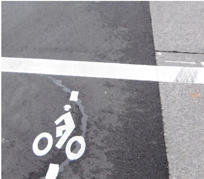
Bicycle Detector Marking at Signalized Intersection
