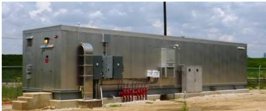
**Figure 2-15 Typical Pressurization Plant**
