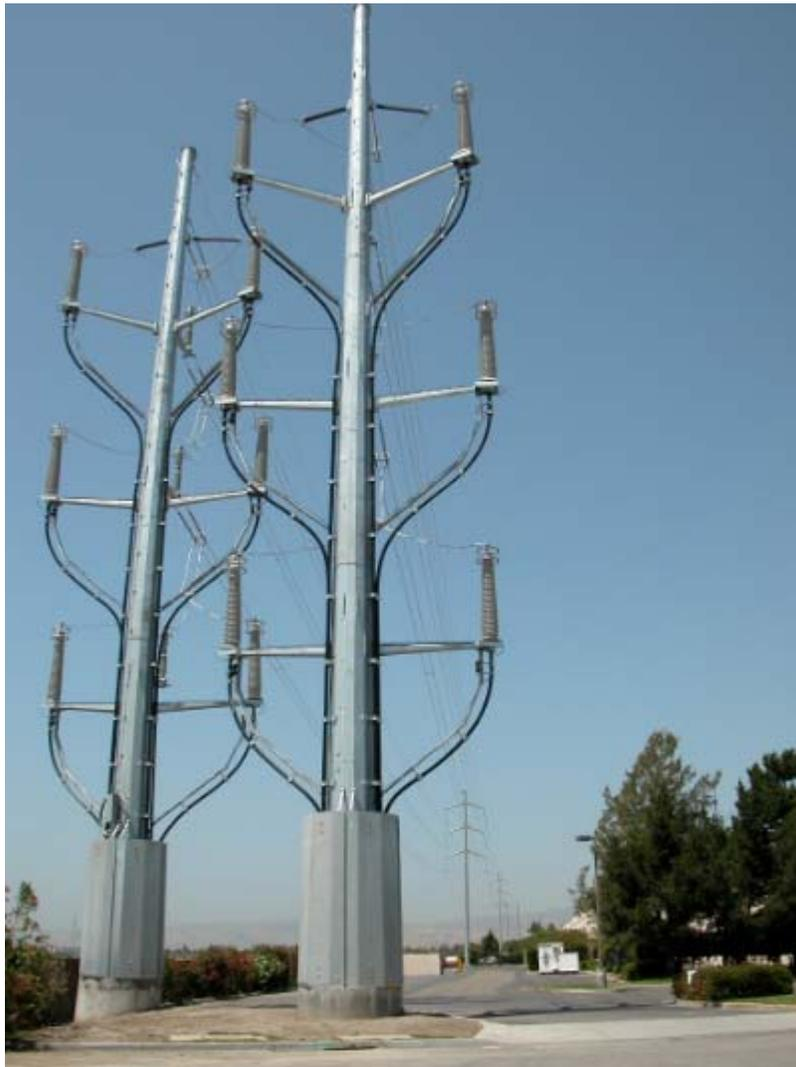
**Figure 3-10 Typical 230 kV Riser Structure**
