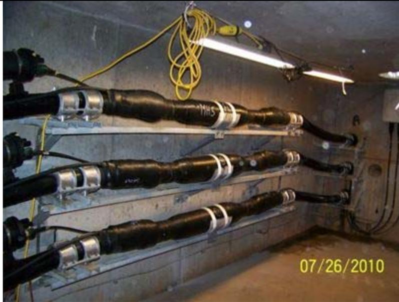
**Figure 2-2 Typical 230 kV Pre-Molded XLPE Splices**
