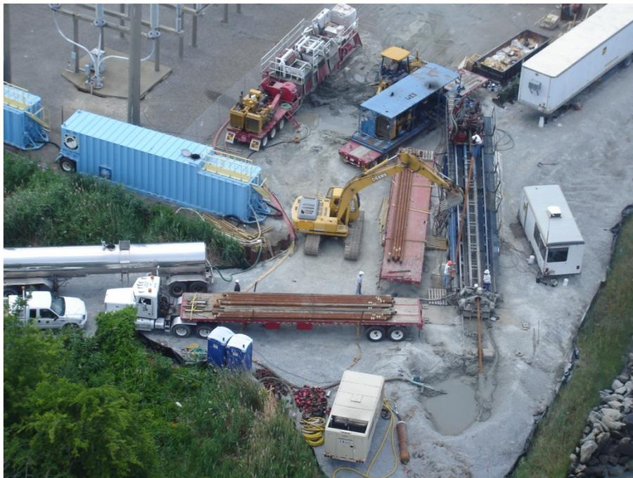
Figure 2-7 Typical HDD Setup
