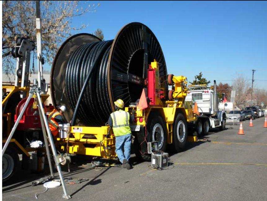
Figure 2-10 Typical Cable Pulling Set up
