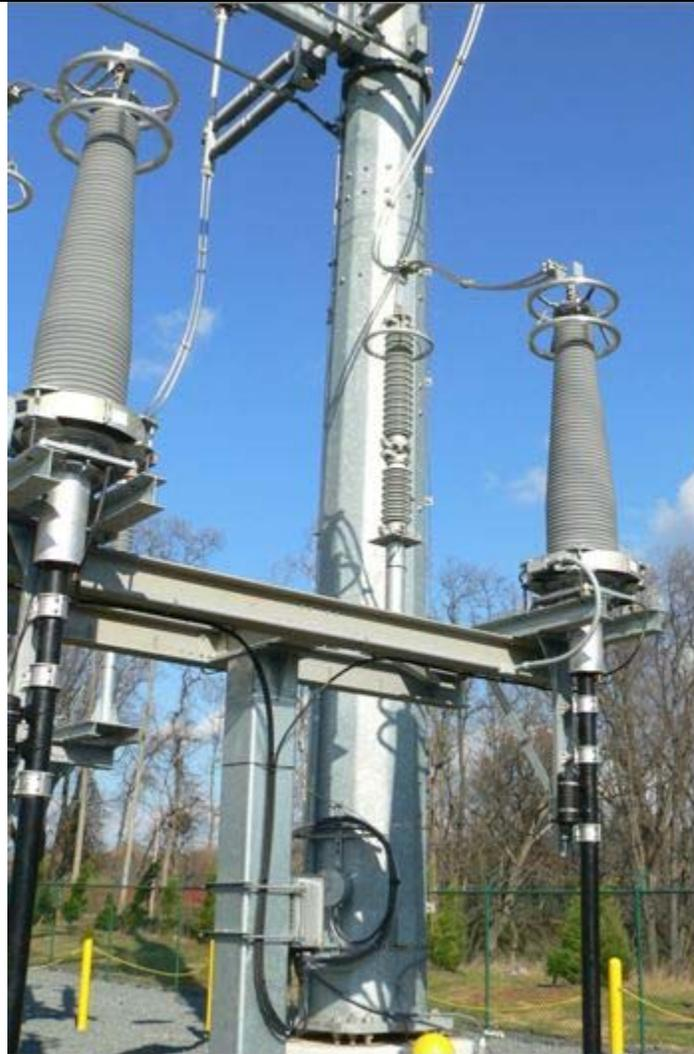
**Figure 2-3 Typical 230 kV XLPE Terminations**
