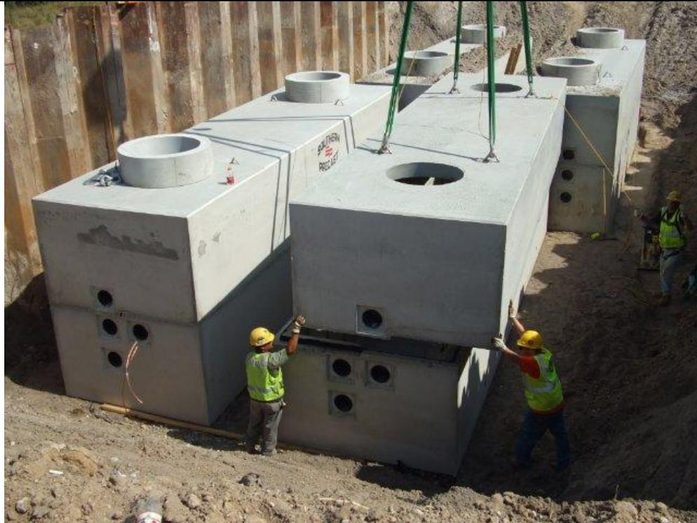
**Figure 2-9 Splicing Vault Installation**
