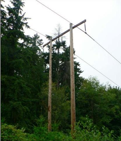
Existing transmission line H-frame structure
