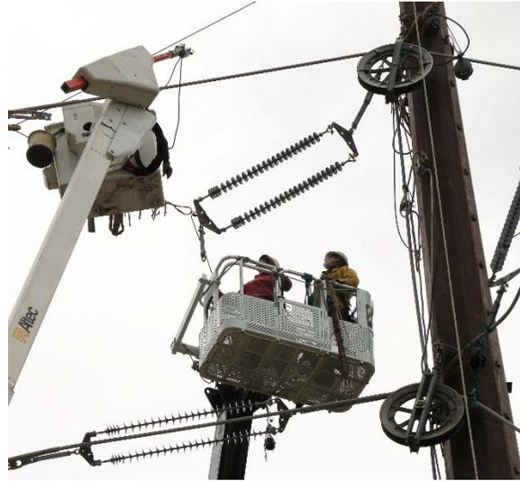
Workers connecting a transmission line to insulators
