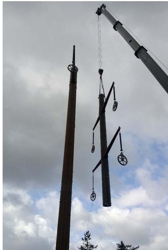
Installing a steel monopole with pulleys attached
