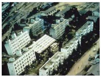
Figure 13. Liquefaction, Niigata Japan, 1964.
