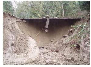
Figure 3. West Lake Sammamish Road Damaged after Landslide in January 2012
