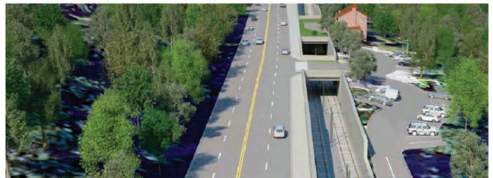
Schematic showing how light rail trains will pass under a lid at the front of the Winters House located on Bellevue Way SE
