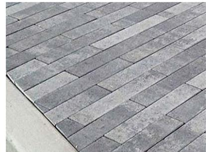
Figure 11 – Permeable Pavers
