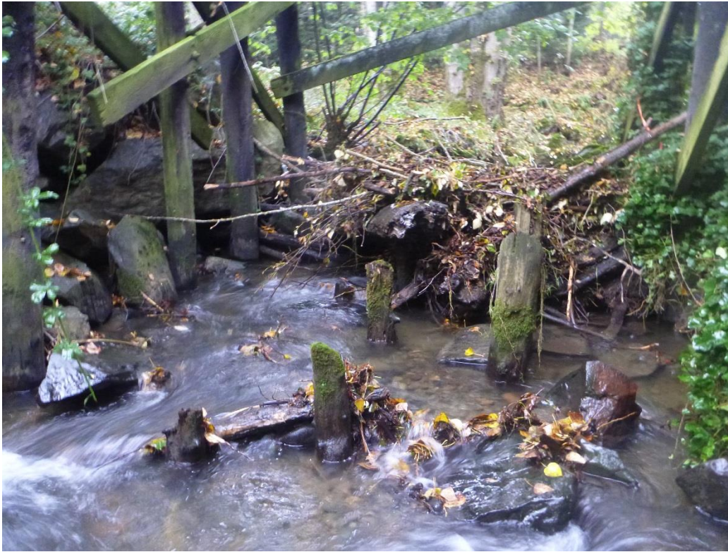
Photo 2: Brush and LWM jammed on pilings under old Northern Pacific Railway trestle (Oct 2013). Some of this debris has been transported downstream as of July 2015 (Scheller, personal communication).
