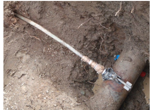
New Service Line and Saddle
