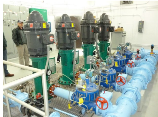
Newport Pump Station Rehabilitation
