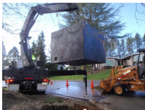
PRV Vault Replacement
