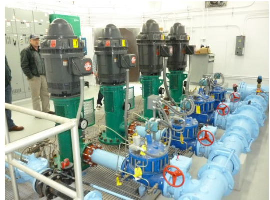
Newport Pump Station Rehabilitation
