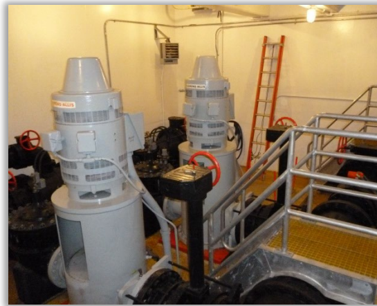
NE 8th Inlet Pump Station
