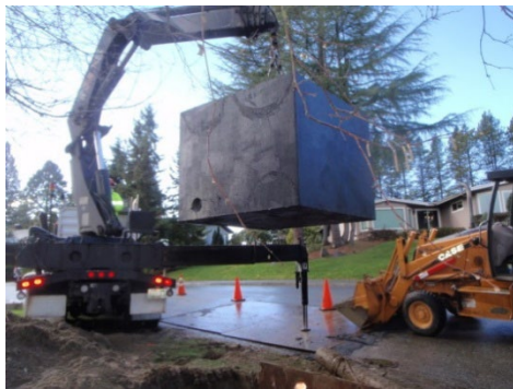
PRV Vault Replacement
