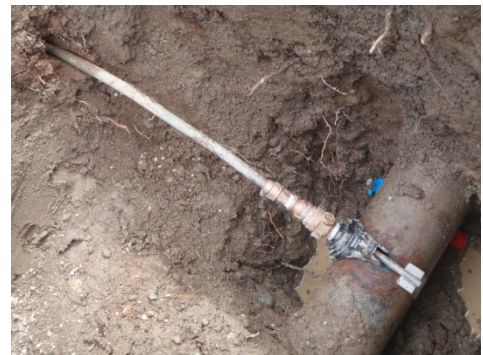
New Service Line and Saddle
