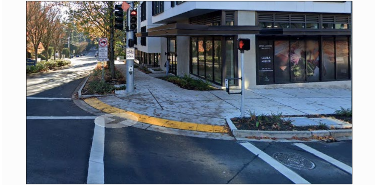
Figure 3-12: Example of Blended Transitions Curb Ramp - Main Street, Bellevue
