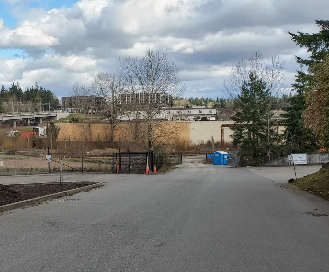
Spring Boulevard at Park
