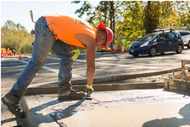
City worker smooths out concrete with trowel.
