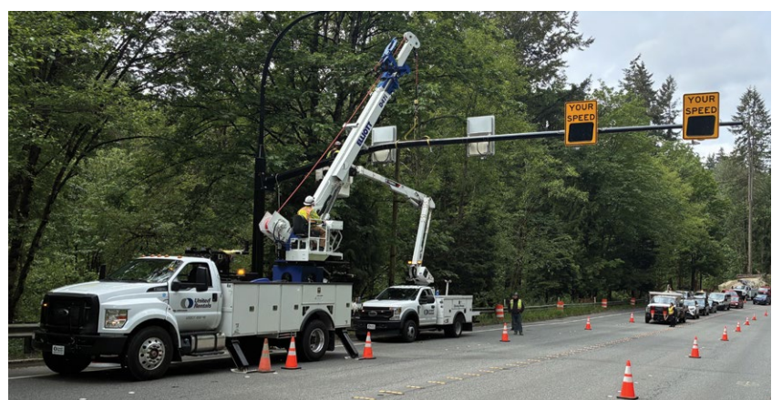
The reduction of the speed limit on a section of Coal Creek Parkway from 40 mph to 35 mph comes with installation of radar feedback signs, which tell drivers how fast they're going.
