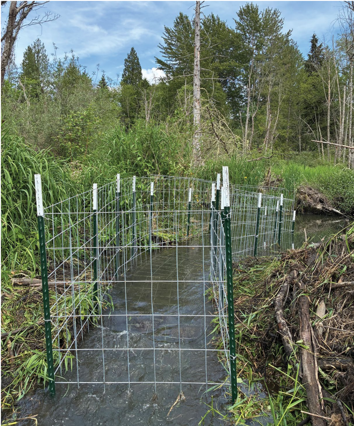
A beaver deceiver in Richards Creek discourages beavers from building dams where they can cause the water level to rise.
