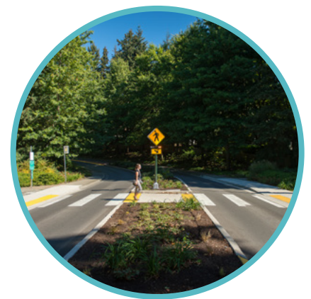
Crosswalk equipped with Rectangular rapid flashing beacons and center refuge island
