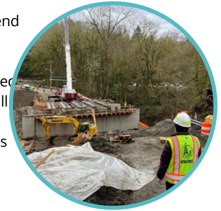
Bellevue Utilities Lakemont Boulevard bridge project to replace a failed culvert
