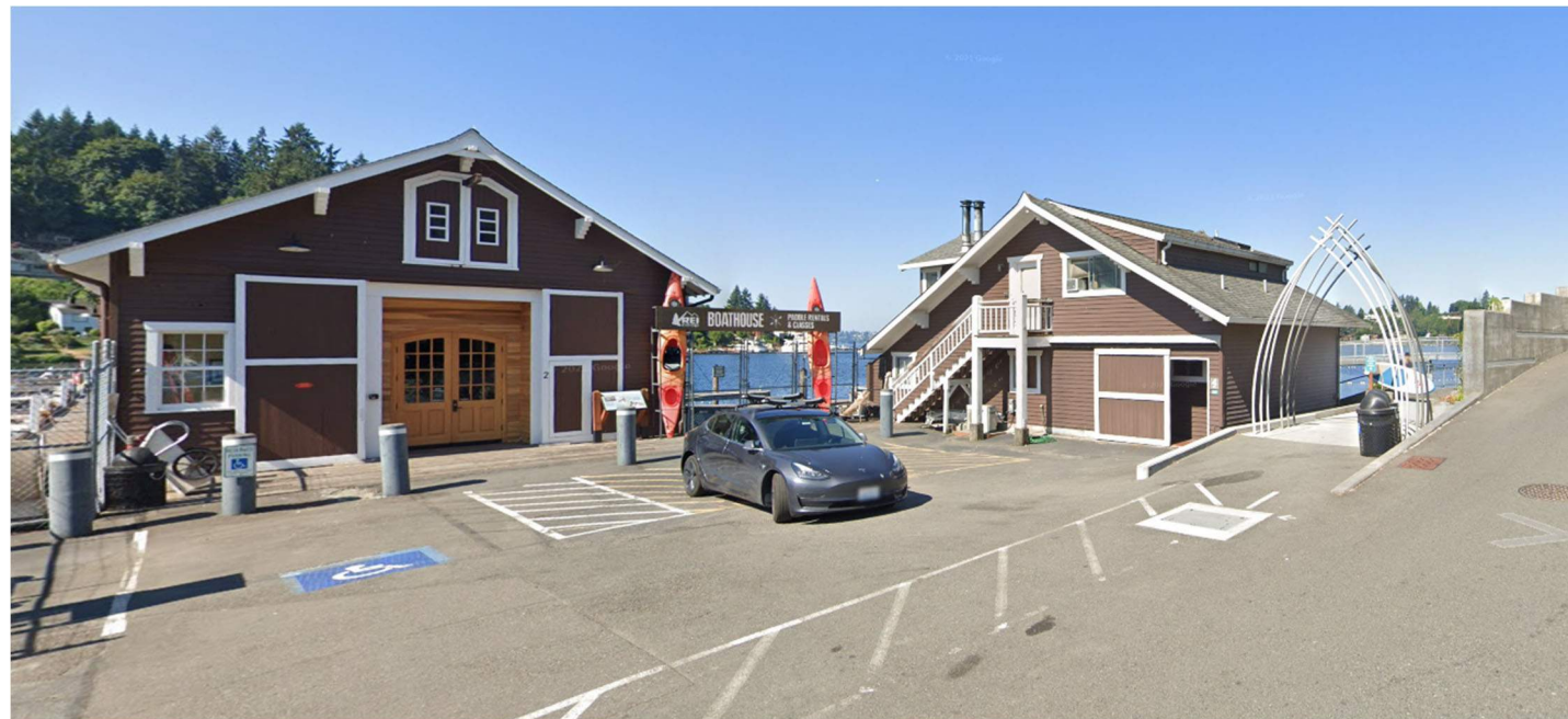
The existing Whaler Building and Ice House. The design goal is to re-envision the Ice House to create a strong pedestrian connection to the beach and the Phase 1 park.
