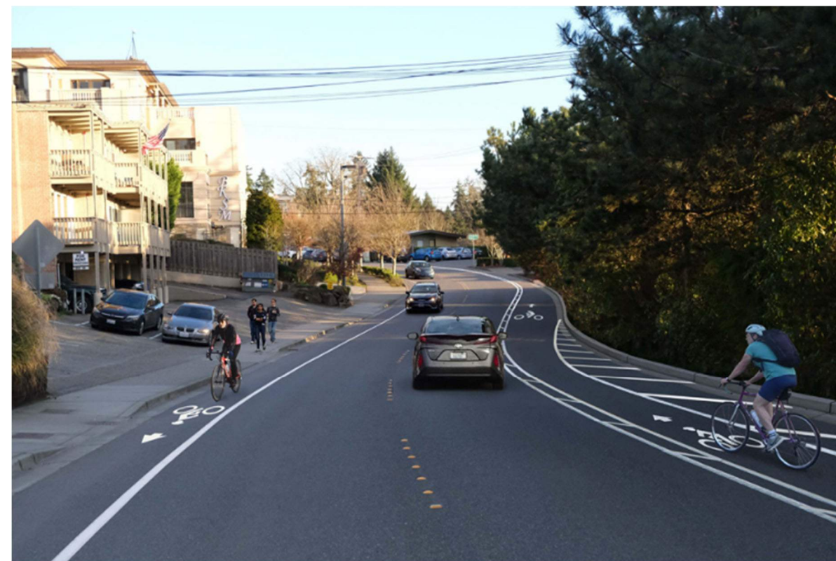
Interim condition being implemented by the city includes adding a bicycle lane to the south edge. This report and the Master Plan explore adding pedestrian infrastructure on the south edge in addition to bicycle infrastructure.
