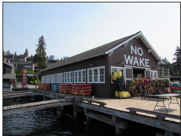
Figure 5-3. Whaling building, view northeast.
