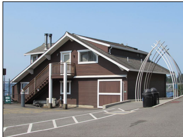
Figure 5-8. Garage, view southwest.
