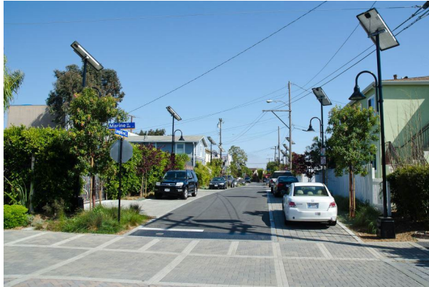
Pavers signal crosswalks, which could be considered where the grade of 100th Avenue shallows out to 2%. Image source: Jarret M, < https://www.vta.org/cdt/street-design-home-page/shared-street-woonerf >
