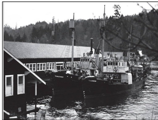
Figure 5-6. Undated photograph showing whaling vessels next to the whaling building, with the main office in the background and the garage in the foreground.
