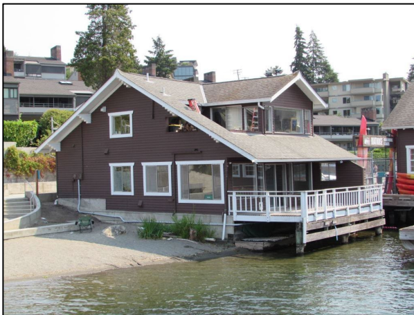
Figure 5-7. Garage, view northeast.
