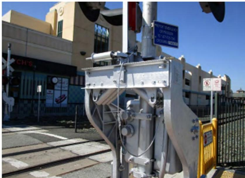
**120.3.1.8** The design of a pedestrian crossing must include pedestrian flashing lights with additional low-mounted flashers and electronic warning bell(s).
