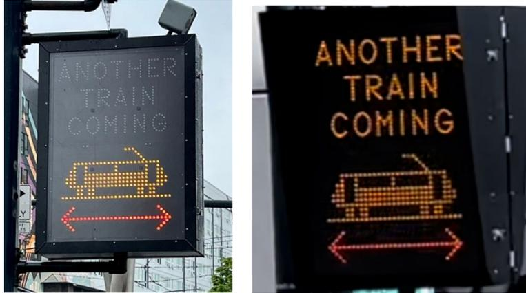
**120.3.2.6.1** At a station platform, the design must include additional pedestrian warning sign(s) at the end of the walkway(s) from station platform to warn passengers exiting the station.
