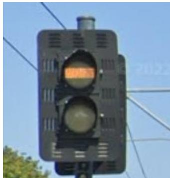
*Commentary: The traffic signal controller for the signalized intersection operates the LRT signals. WAC 468-95-365 Light Rail Transit Signals states the following:*
