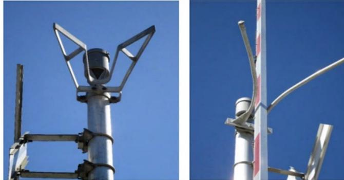
**120.3.1.7.13** The DOR must design the crossing to include gate keeper assemblies.
