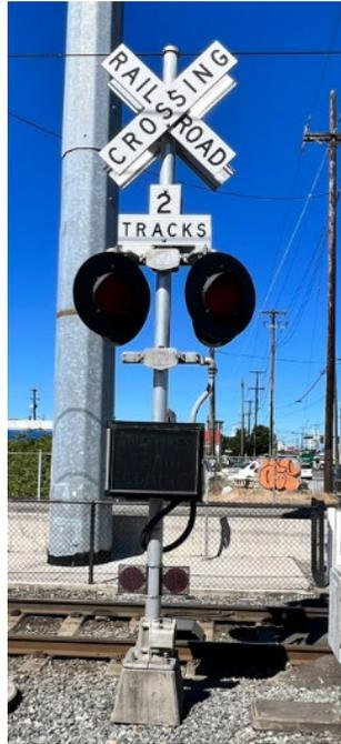
**120.3.1.8.1** When the pedestrian crossing is part of a roadway crossing, then pedestrian flashing lights must flash in unison with the roadway flashing lights.
