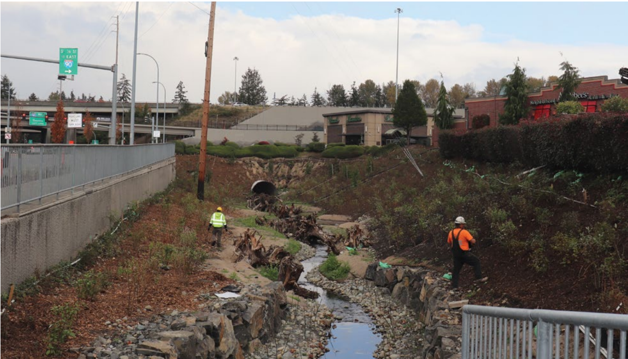
A major project in Factoria completed last year involved installation of a concrete holding tank under Factoria Boulevard and channel improvements to Richards Creek.
