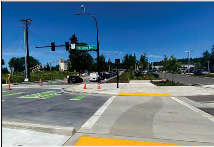
Intersection of 130 th Ave NE and NE Spring Blvd. The subject is located at the northeast corner of the intersection, north of the BelRed/130 th Street Sound Transit Station.
