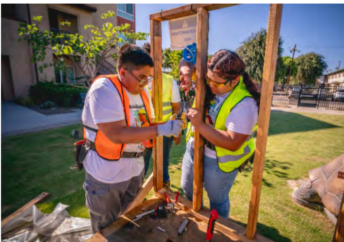
BRIDGE partnered with Harbor Freight Tools for School to train local teens in construction trades at Jordan Downs, Los Angeles
