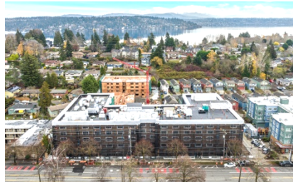
The Flourish on Rainier under construction
