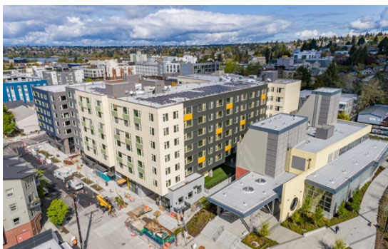
Cedar Crossing in Development — View from Southeast with Roosevelt station entrance to the right
