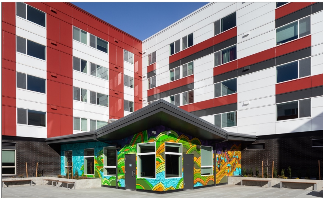
Flourish on Rainier, completed 2023
