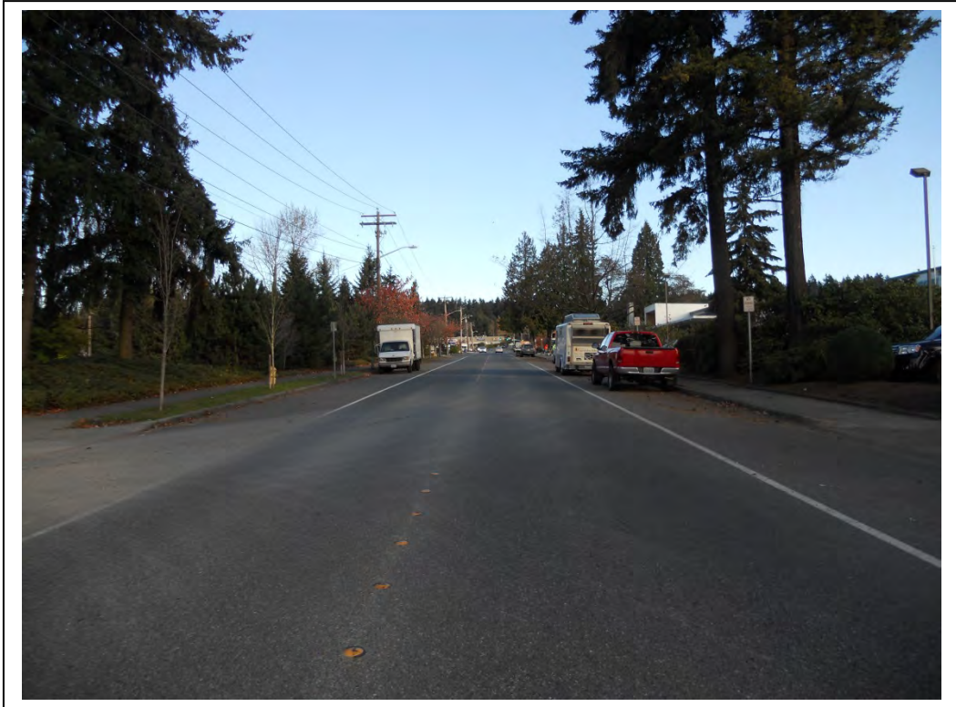
Photo 15: 130 th Avenue NE, facing north.
