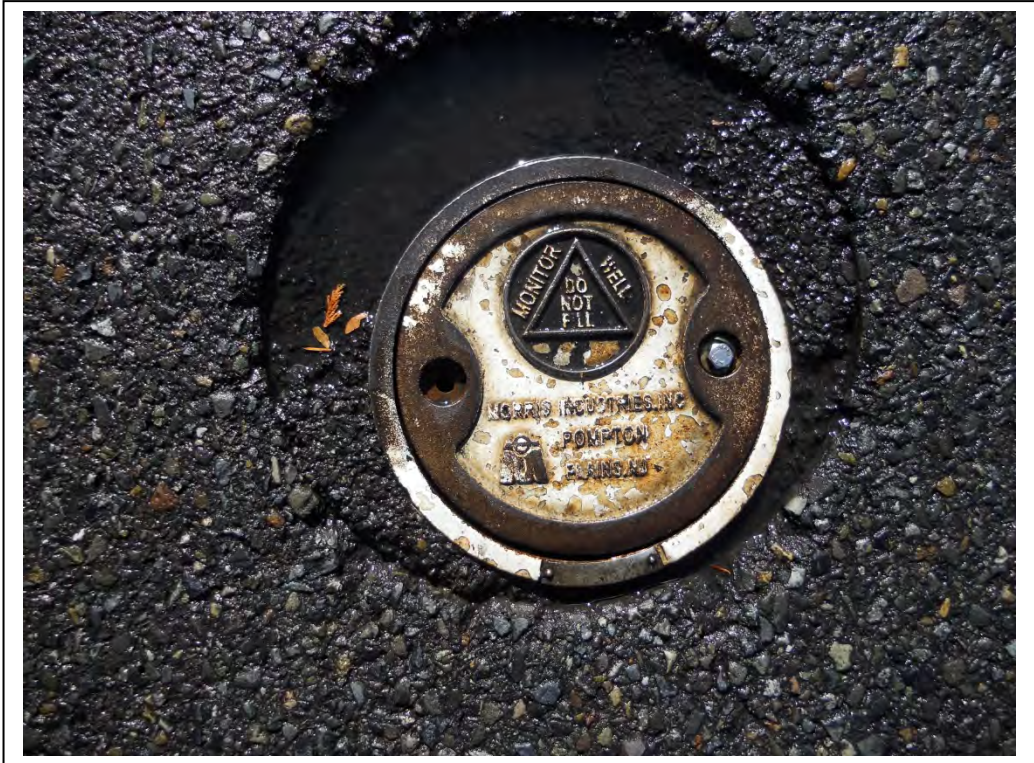
Photo 21: Groundwater monitoring well (E340-B-019) in 130 th Avenue NE, adjacent to the southwest of the subject parcel.
