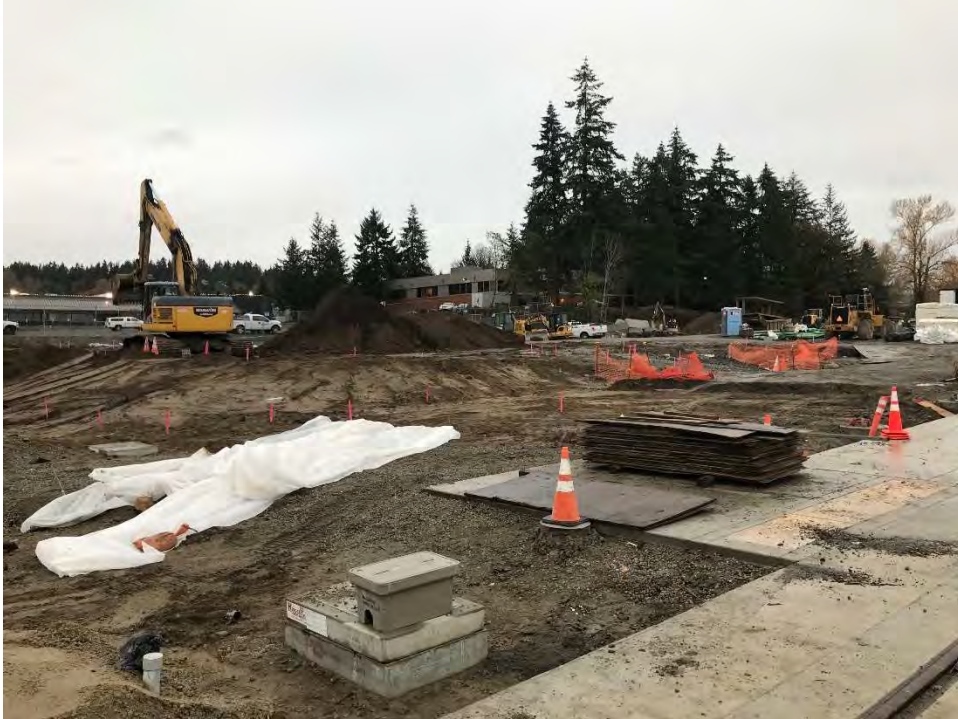
Photo 1. Overview of current conditions at the site.
