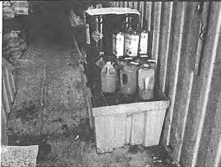
PHOTO #5: CHEMICALS STORED INSIDE CONEX HAVE SECONDARY CONTAINMENT
