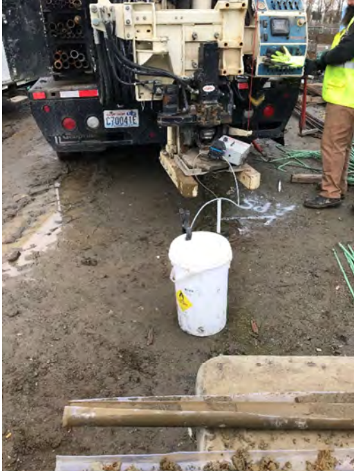
Photo 7. Groundwater sampling of Borehole B23
