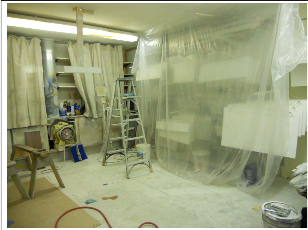
Photo 13: Paint booth in The Wall Doctor, Inc. space, looking south.
