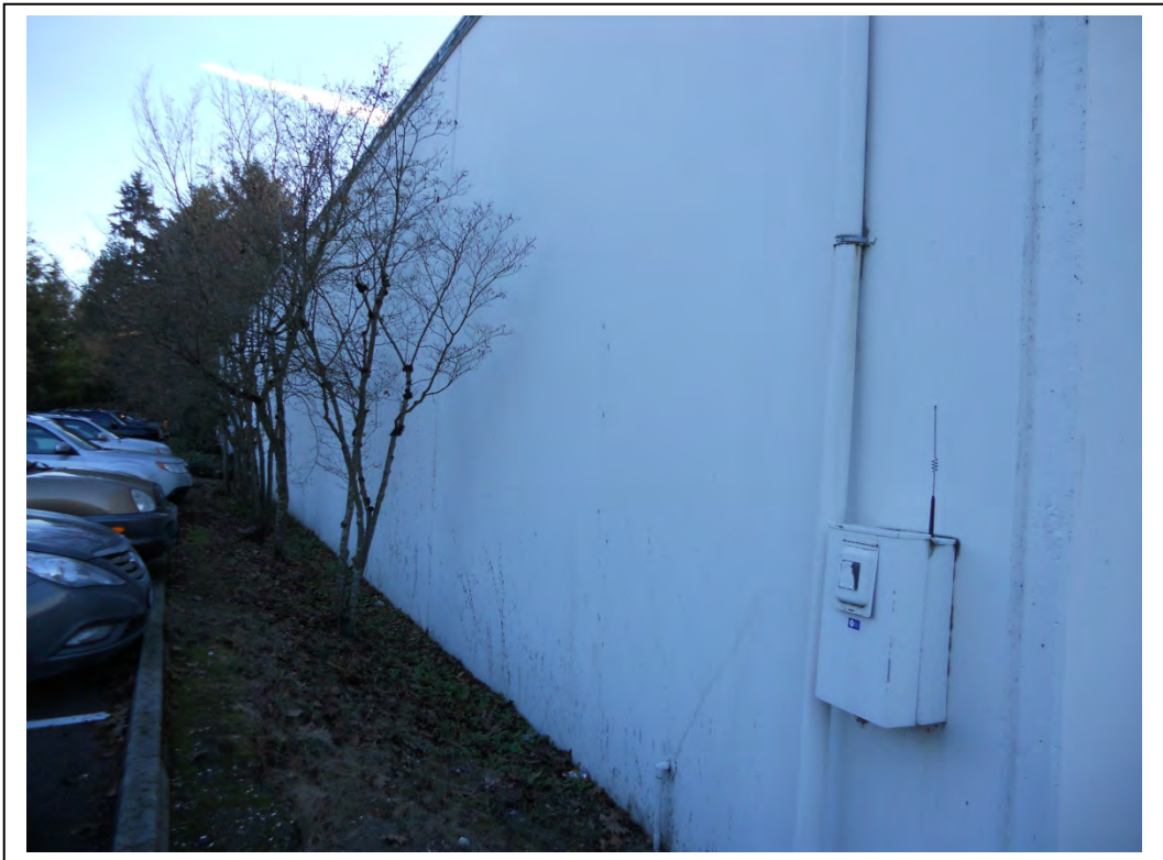
Photo 3: Facing southeast towards north exterior of subject office building.
