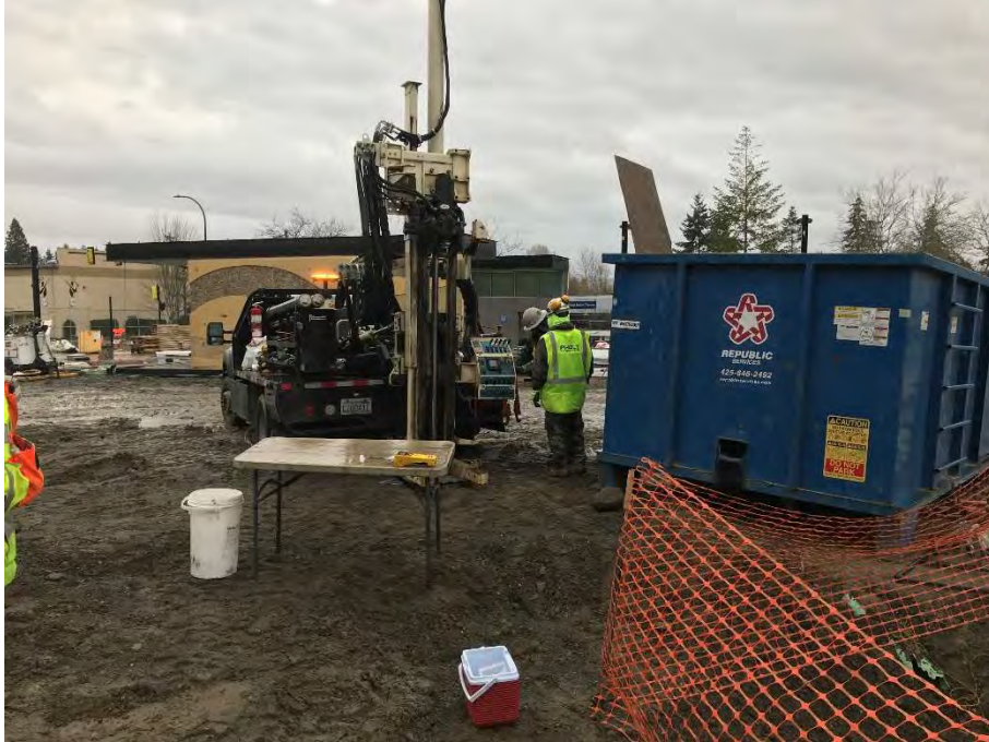
Photo 13. Overview of Borehole B26
