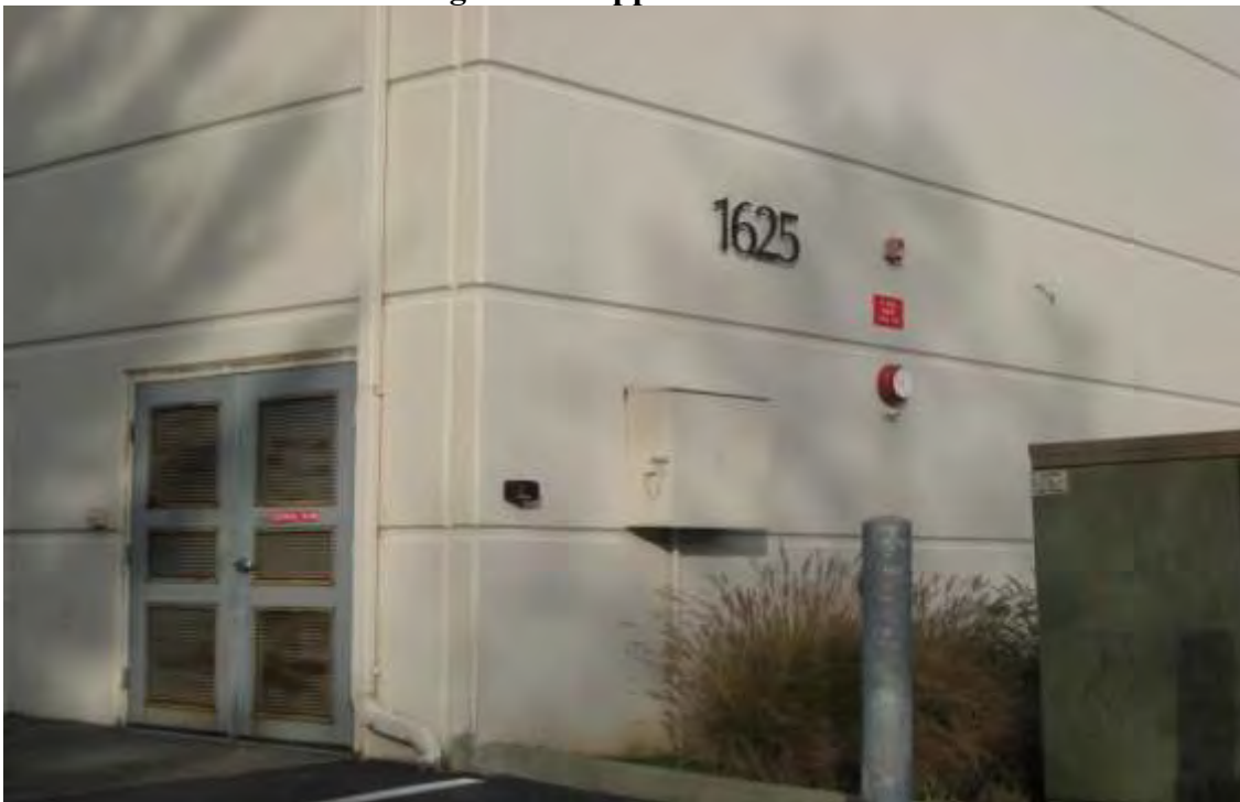
Photo 4: South Side of the Building – near capped contamination
