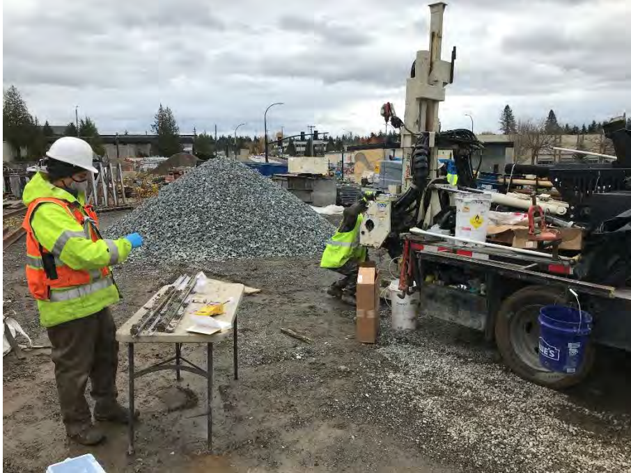
Photo 9. Drilling of Borehole B24
