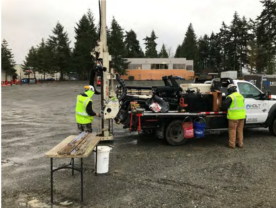
Photo 17. Drilling of Borehole B28
