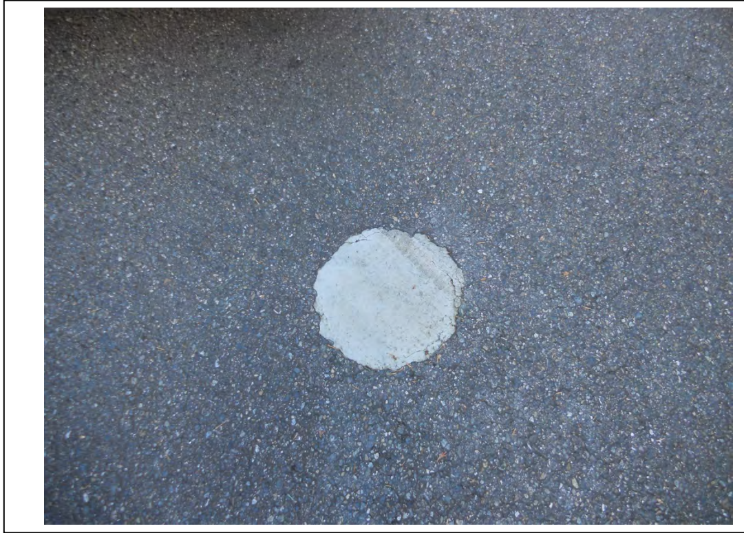
Photo 10: Capped soil boring noted in southeast parking area of subject parcel (refer, Figure 2).
