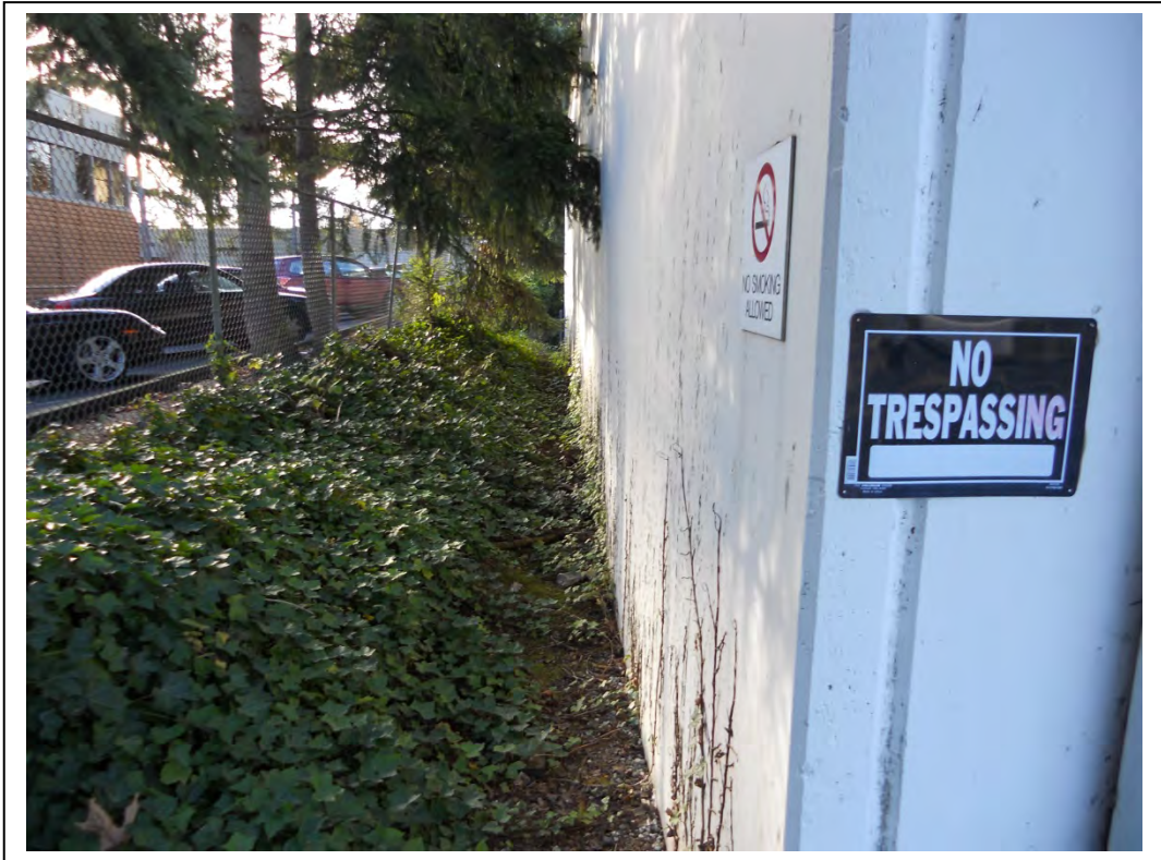
Photo 4: Looking south at the east exterior of the subject building.
