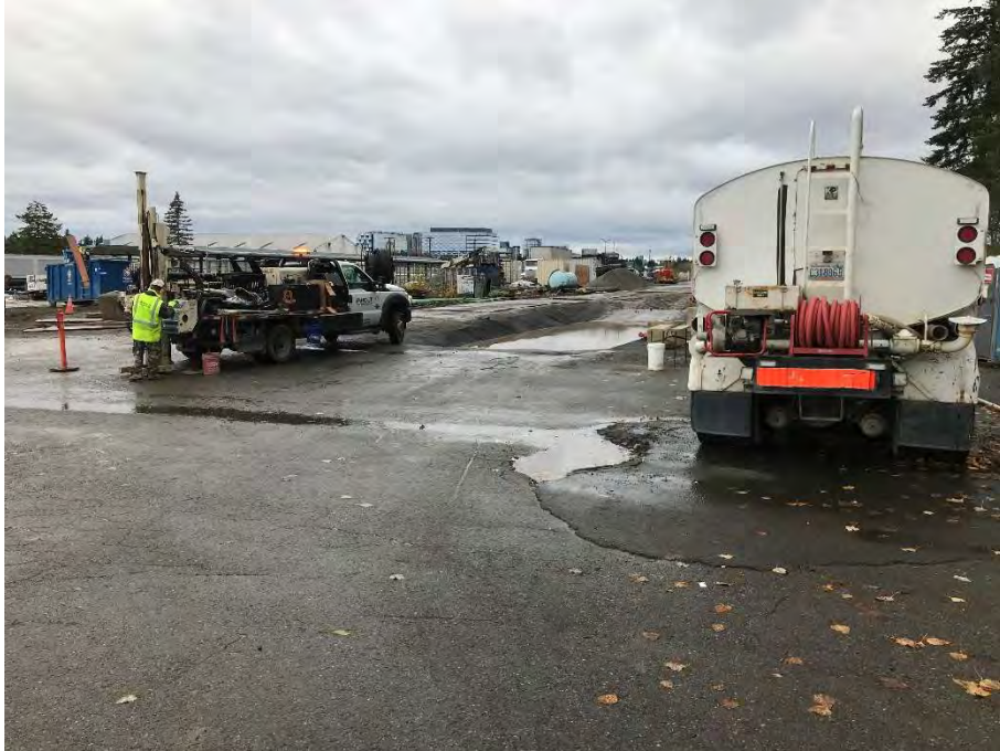
Photo 11. Location of Borehole B25
