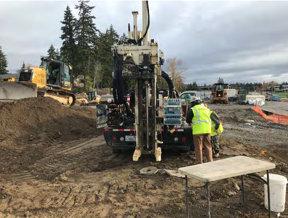
Photo 3. Drilling at Borehole B21.
