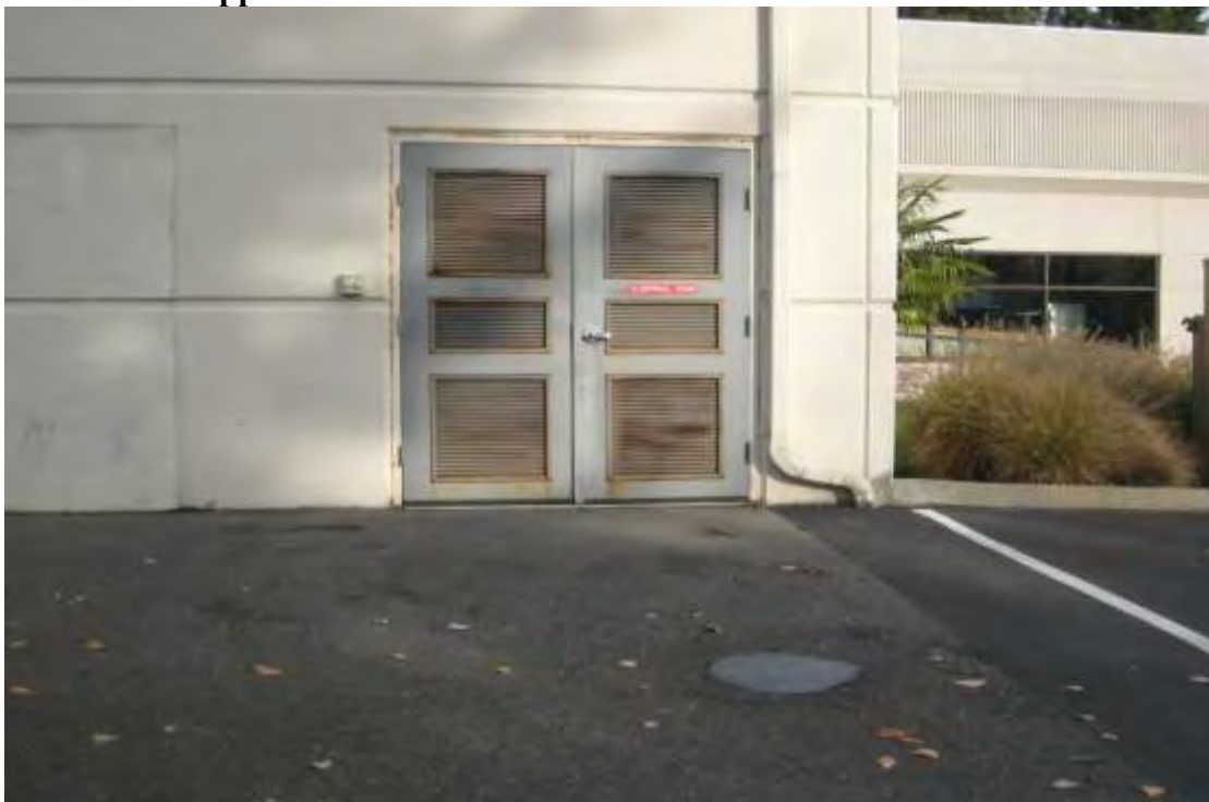
Photo 2: Area of capped contamination - from the south
