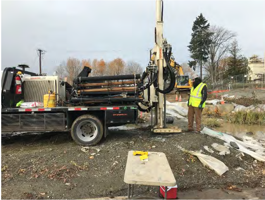
Photo 5. Location of Borehole B22
