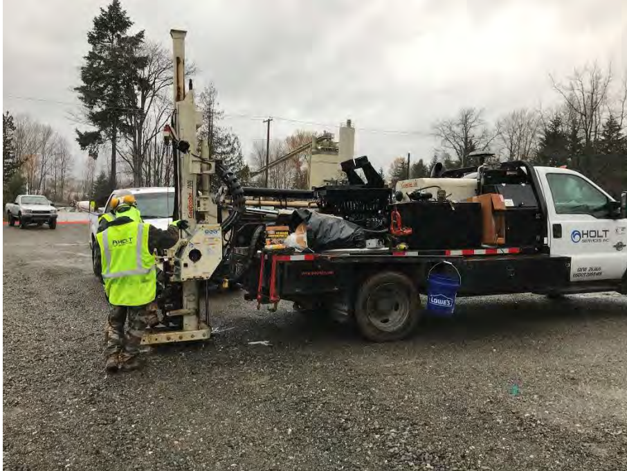
Photo 15. Drilling of Borehole B27
