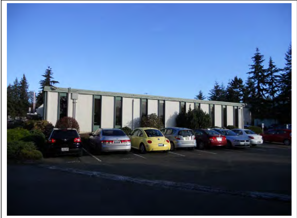
Photo 2: Looking north at the south exterior of the subject office building.
