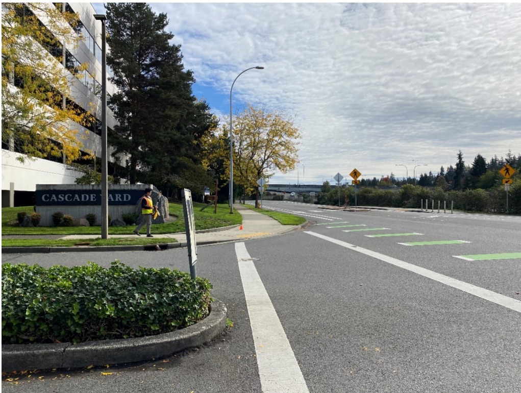
View looking east on SE Eastgate Way (pedestrian sight distance) at 146 th PI SE.
