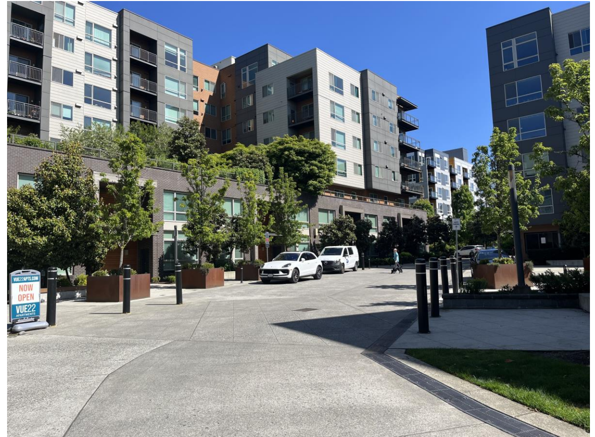
NE 22 nd Pl between Bel-Red Rd and 156 th Ave NE Vue 22, Bellevue
