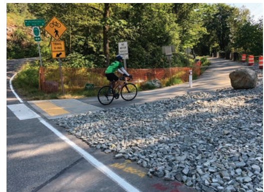
4 Bollards with boulders prevent entrance to the multipurpose path by unauthorized motor vehicles
