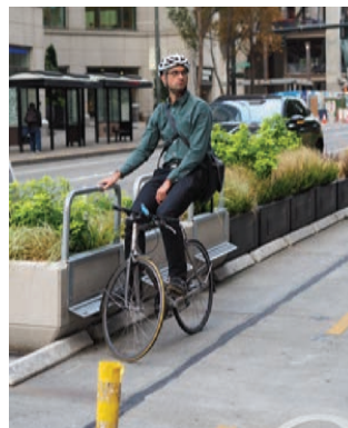
3 Lean rail and planter buffer along protected bike lane
