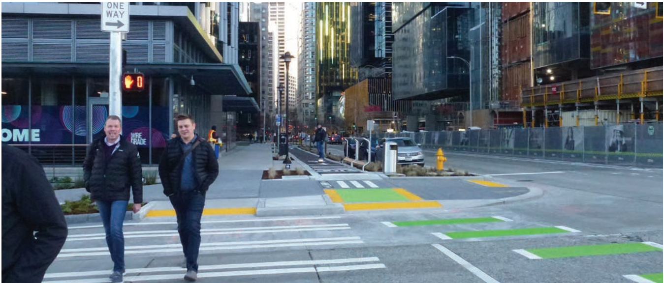
1 Physically separated bikeway and sidewalks meet at the intersection corner.
