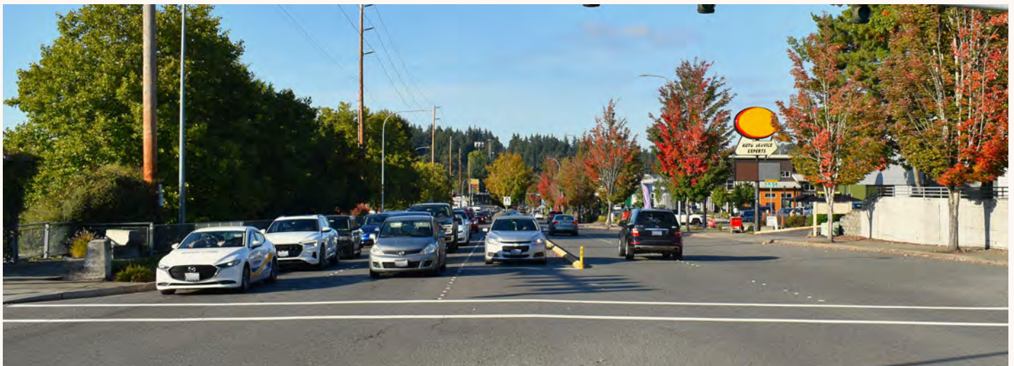
Figure 18: Factoria Boulevard Southeast provides an example of an Urban 35 mph arterial.
