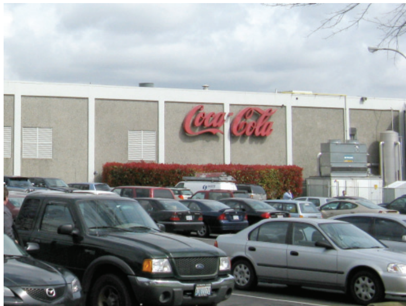
Existing light industrial use.
