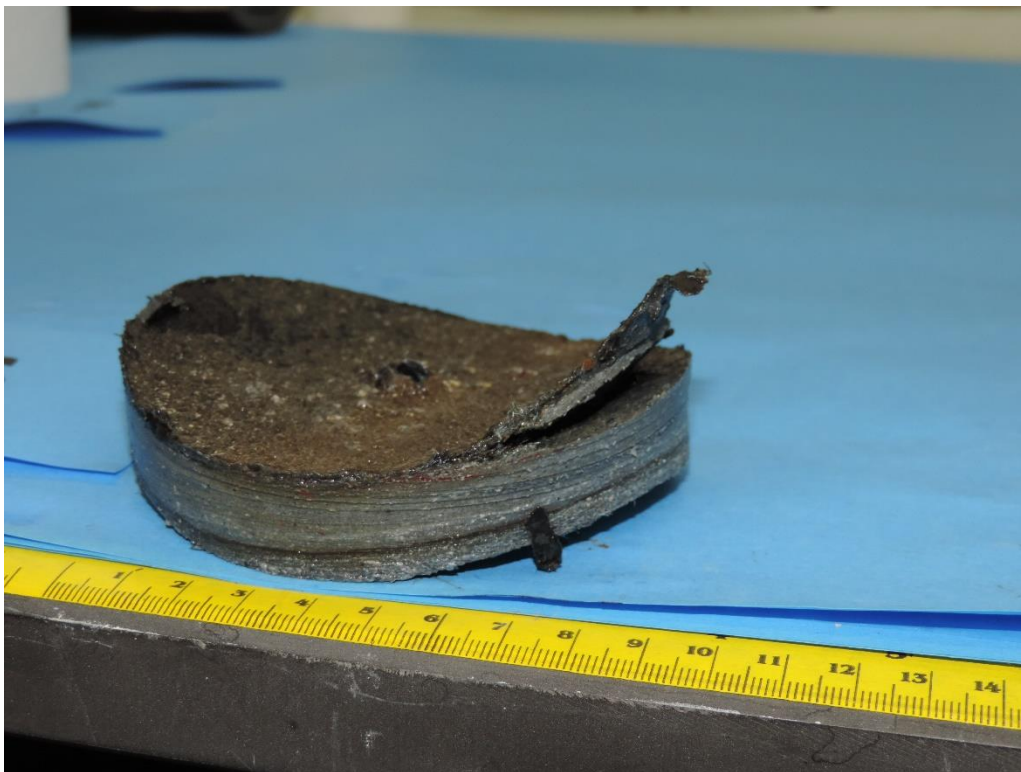
Close up of an area of delamination at the inside layer of N-5.
