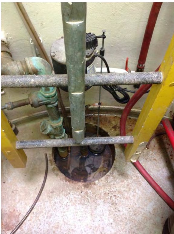
End of ladder, above/adjacent to sump pump and drain
