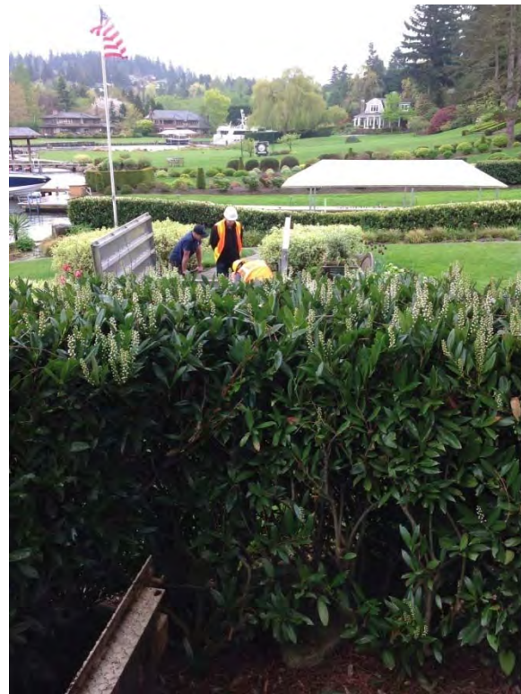
Overall aesthetic top cover vault located in yard
