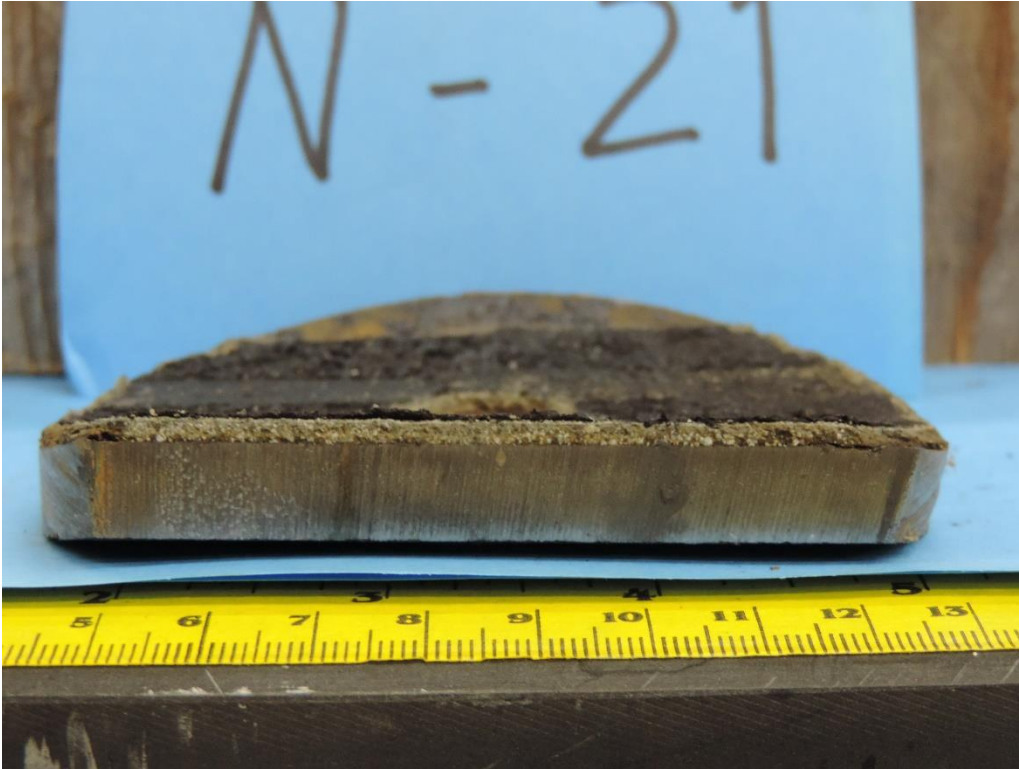
Cross section of sample N-21 after pH and phenolphthalein sampling. That indicated that the cement was slightly acidic.
