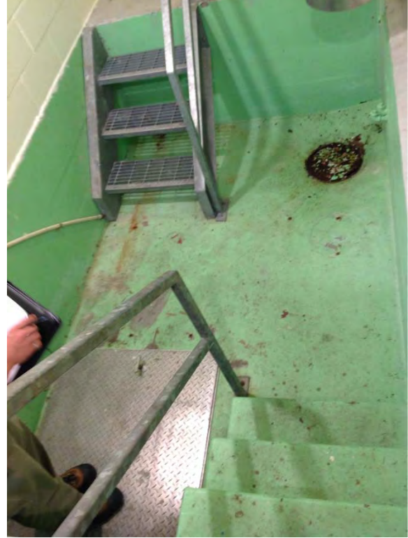
Wet well access hatch
