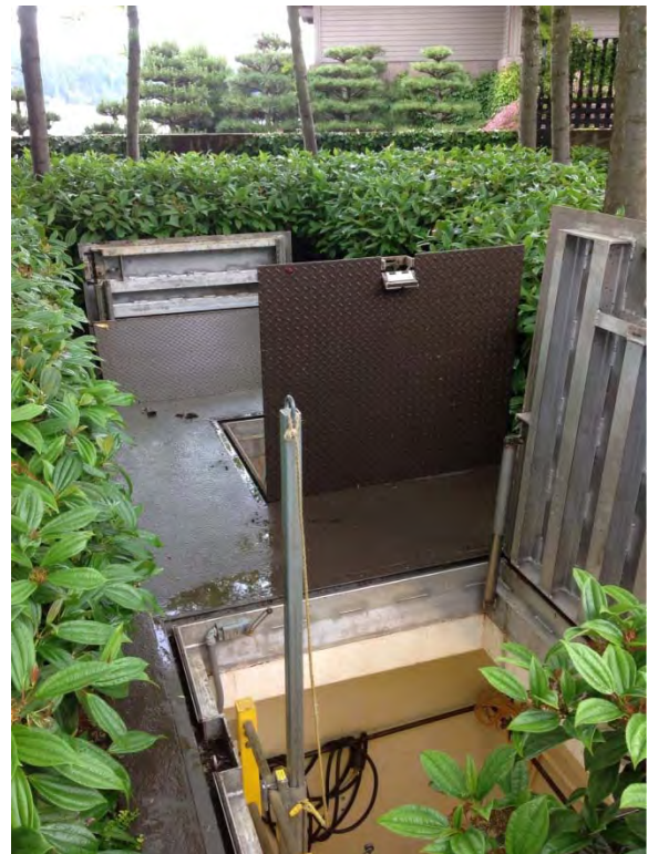
Narrow access around dry pit hatch
