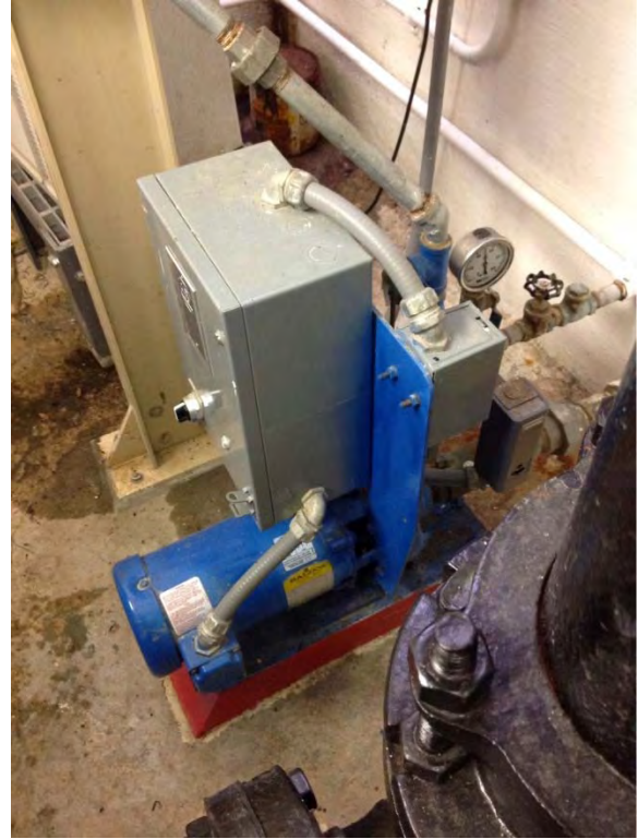
Booster package for water service, water supply from lake
