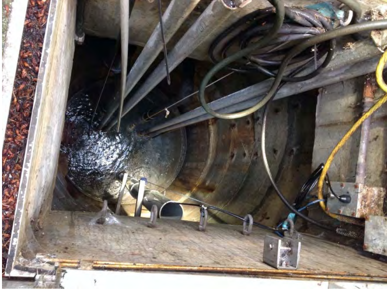
Submersible station, unable to observe pumps
