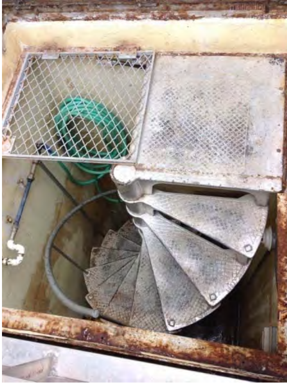
Spiral staircase to dry pit, metal grating used to step onto main platform
