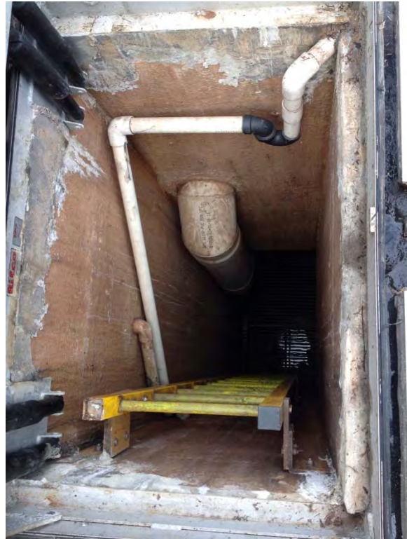
Interior of wet well
