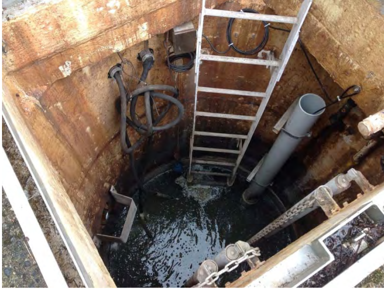
Submersible station, unable to observe pumps
