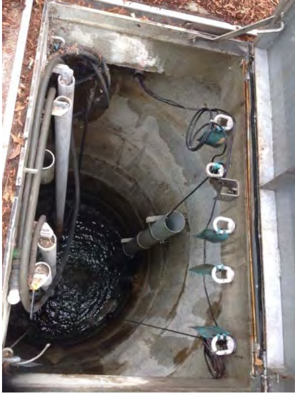
Submersible station, unable to observe pumps
