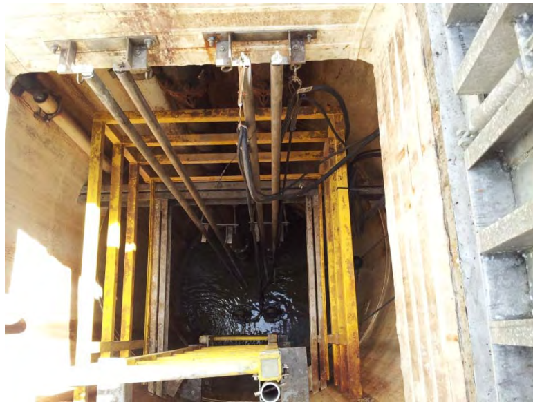
Interior of wet well
