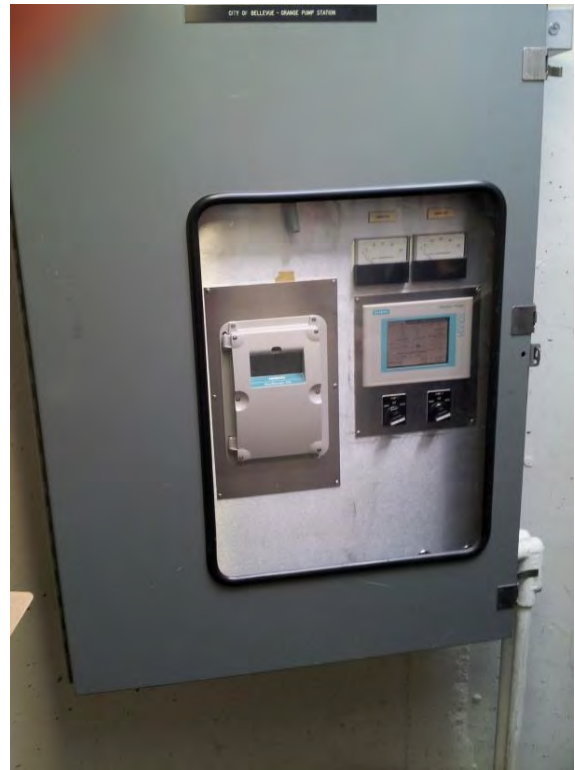
Starters located in dry pit, appears to be in good condition but have decreasing useful life
