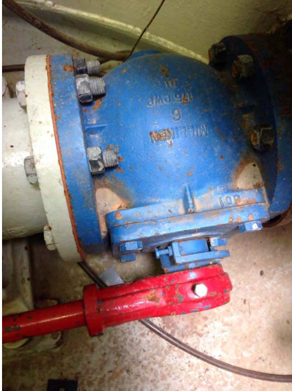
Plug valve horizontal axis of rotation - ideal
