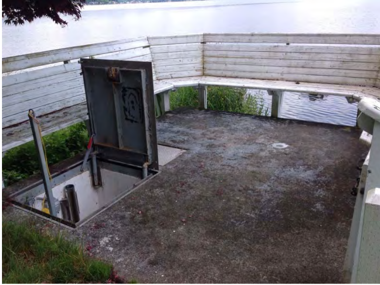
Dry pit access hatch and ladder
