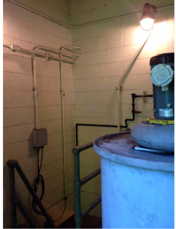
Interior of room above wet well
