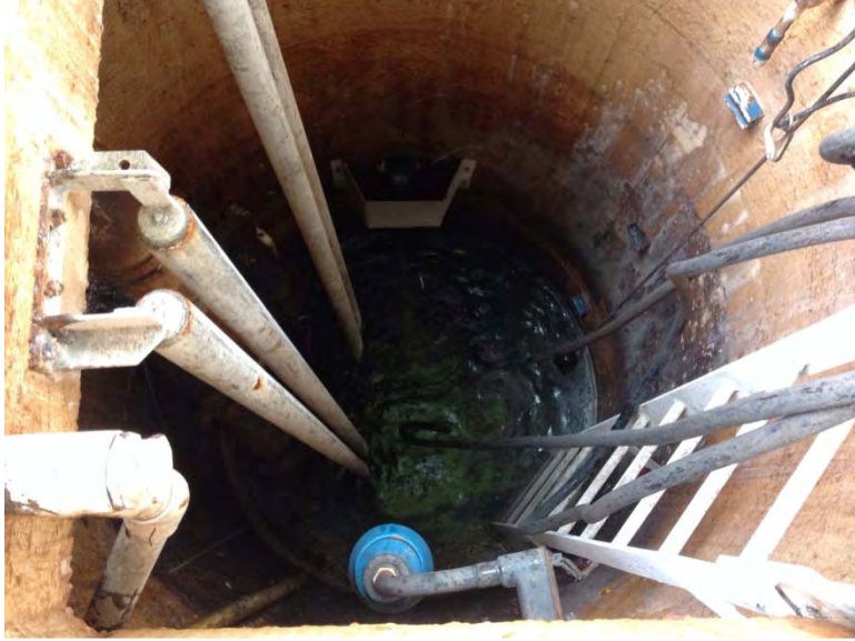
Submersible station, unable to observe pumps
