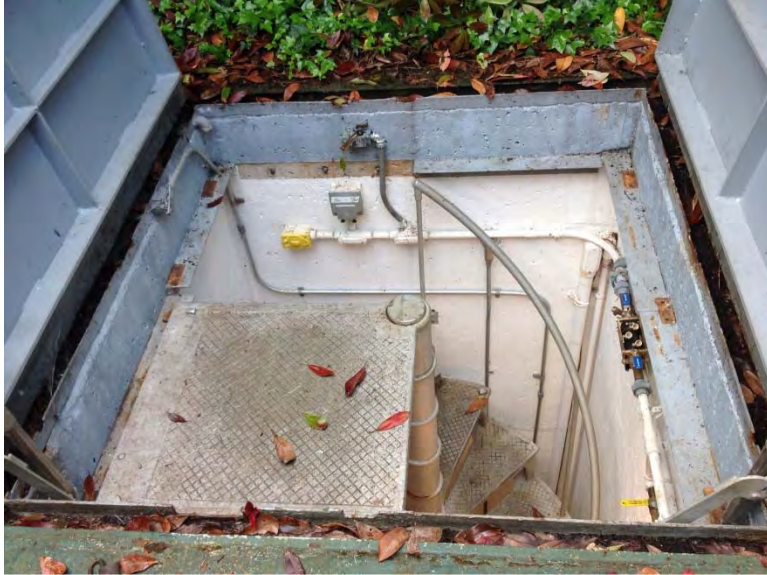
Some new paint interior near hatch and opening
