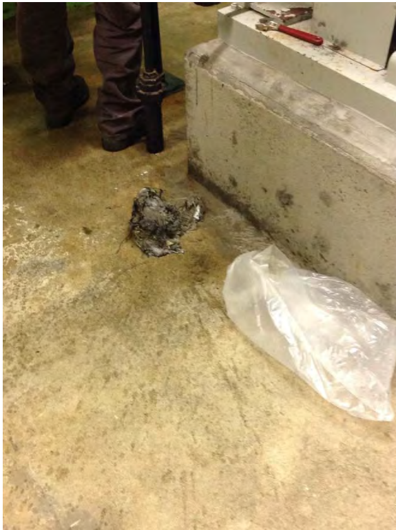
Removal of rags upon site visit
