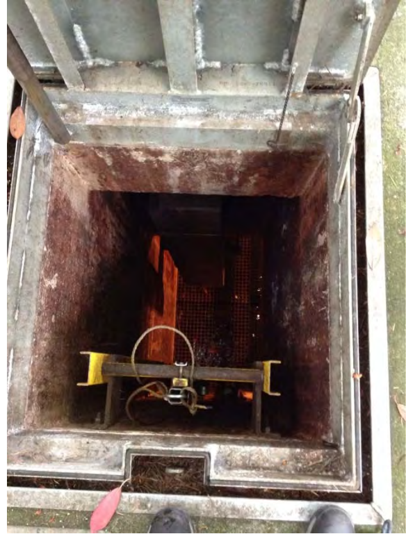
Interior of wet well
