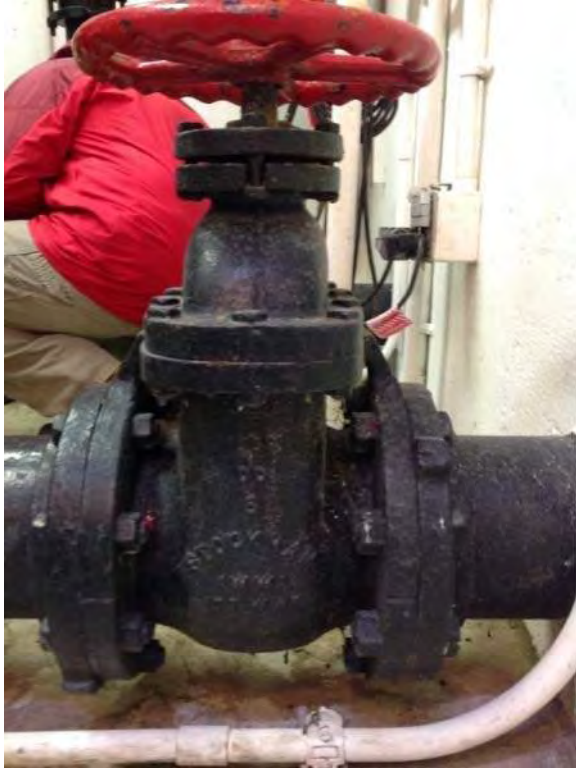
Gate valve isolation for suction piping
