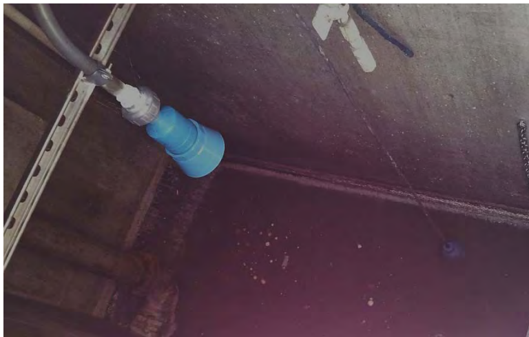
Interior of wet well appears to be in good condition
