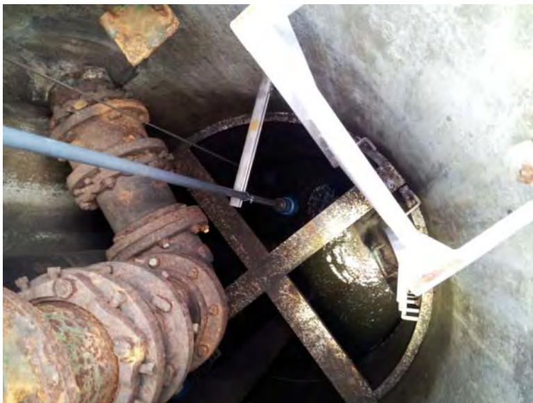
Some sections of grating platform in corner of site
