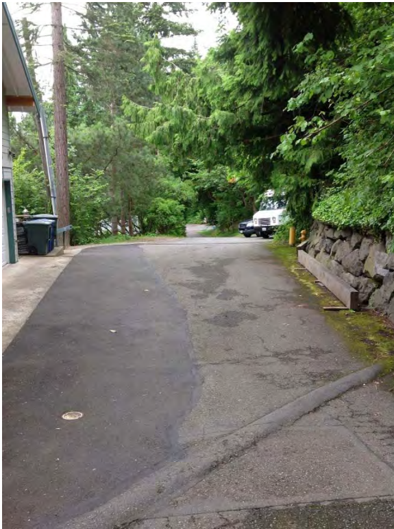
One lane paved road above station
