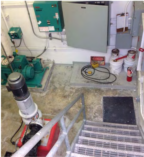
Interior of dry pit appears to be in good condition
