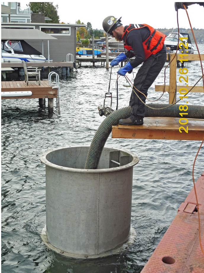
Figure 5.7 City of Renton Emergency Lake Line Cleaning - Temporary Caisson Access
