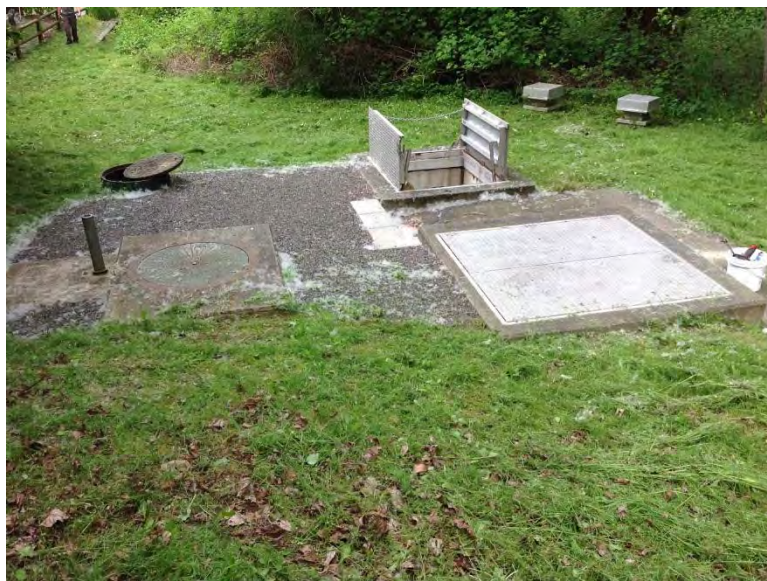
A lot of grass surrounding station, City mows area
