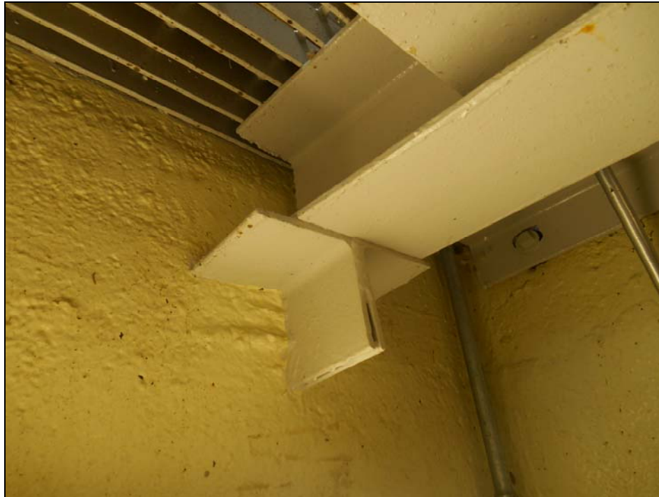
Photo 1: Beam Seat in Good Condition
