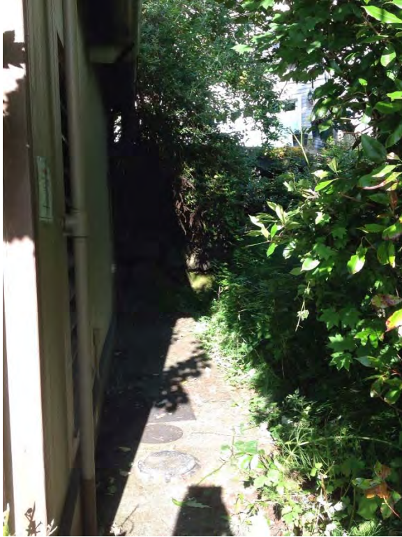
Path to wet well access adjacent to control building
