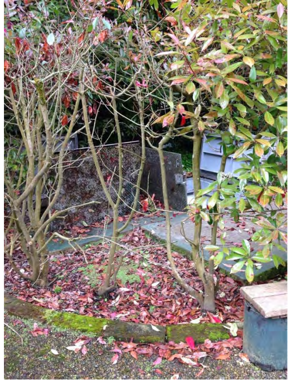
Laurel bushes around surround station to obscure view of vault hatches
