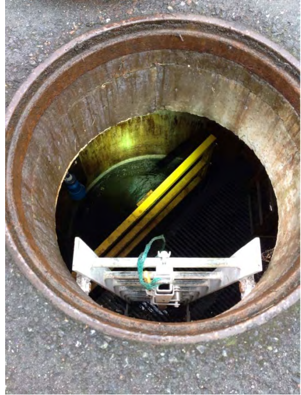
Interior of wet well
