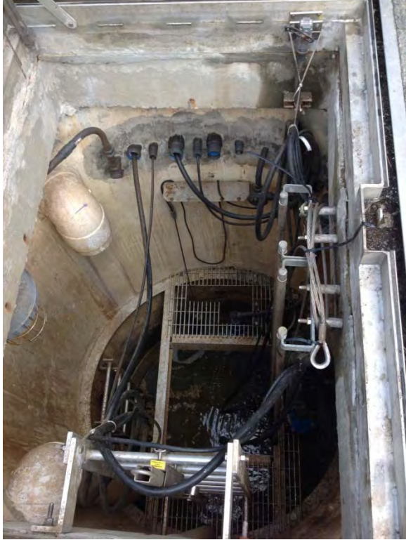
Interior of wet well
