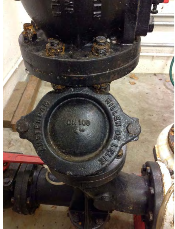
Ball check valve, vertical orientation
