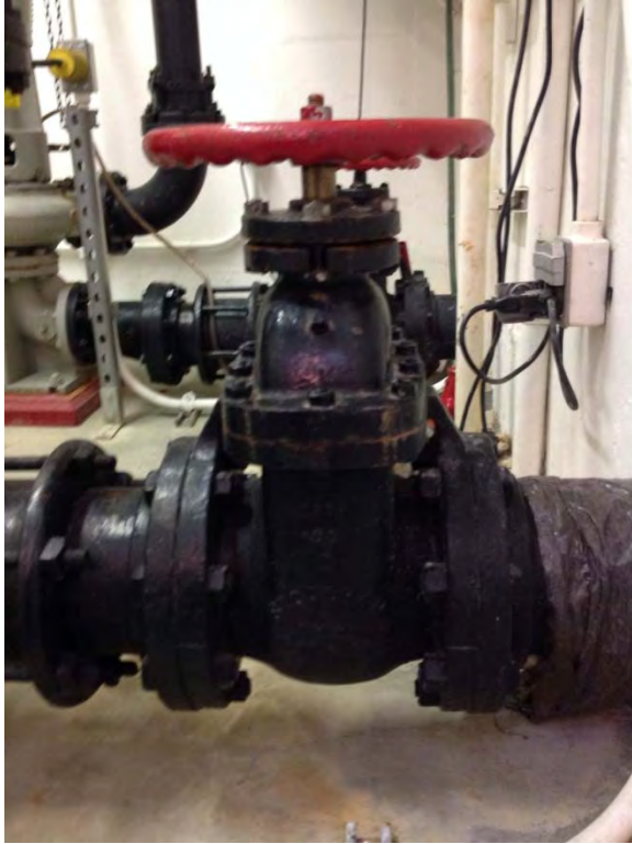
Gate valve isolation for suction piping
