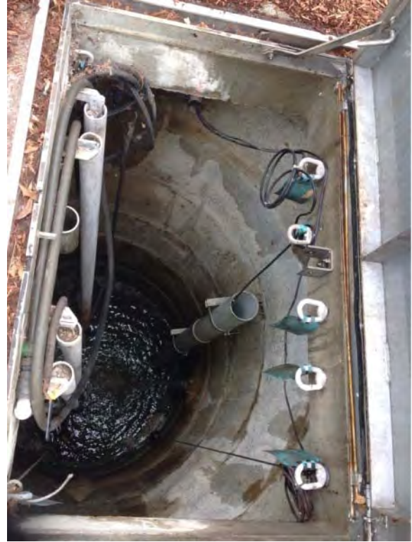
Interior of wet well appears to be in good condition
