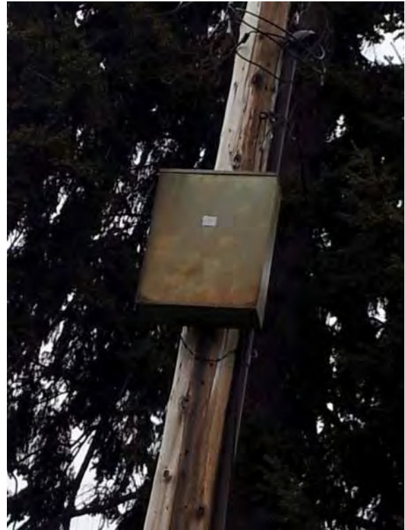
Rusted telephone network interface termination box, located overhead at top Qwest pole
