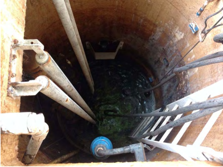
Submersible station, unable to observe pumps
