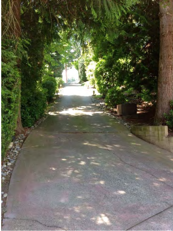
One lane steep driveway access to station
