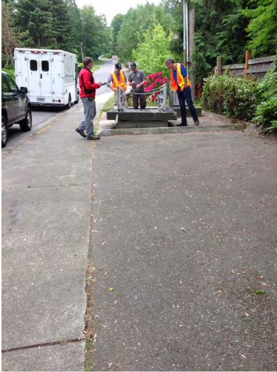
Curb ends adjacent to sidewalk – potential tripping hazard for public
