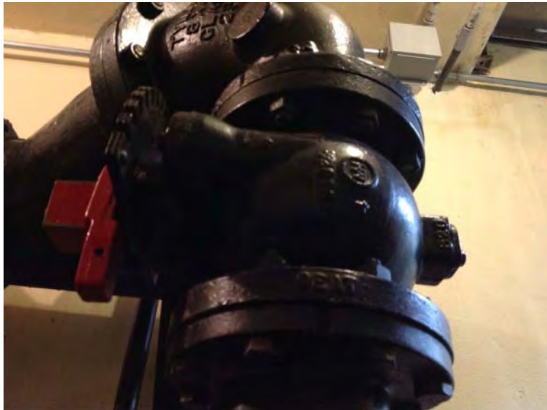
Discharge plug valve
