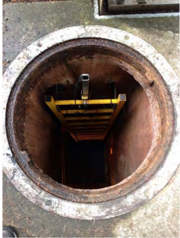
Interior of wet well
