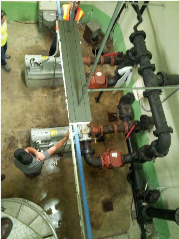
Interior of dry pit
