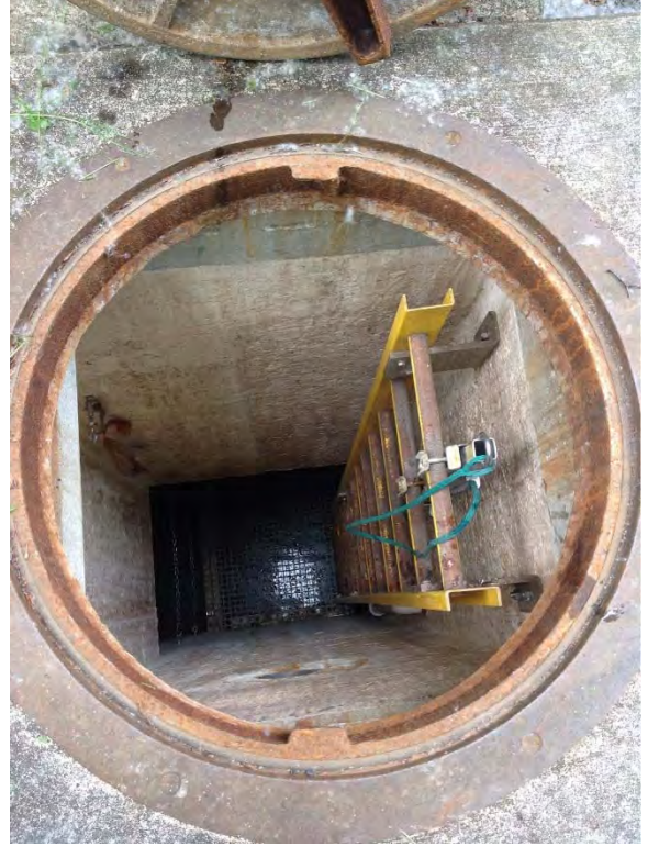
Interior of wet well
