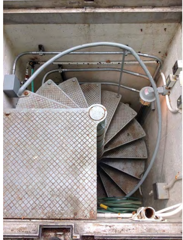
Spiral staircase rail begins at top of staircase
