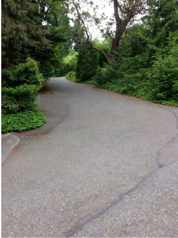
Steep driveway, switch back pavement driveway
