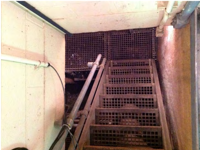
Stairs to access wet well
