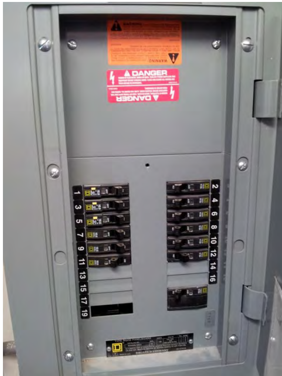
Panelboard located in dry pit, appears to be in good condition, but have decreasing useful life
