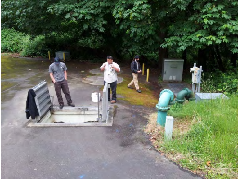
Service meter located on outdoor rack adjacent to station
