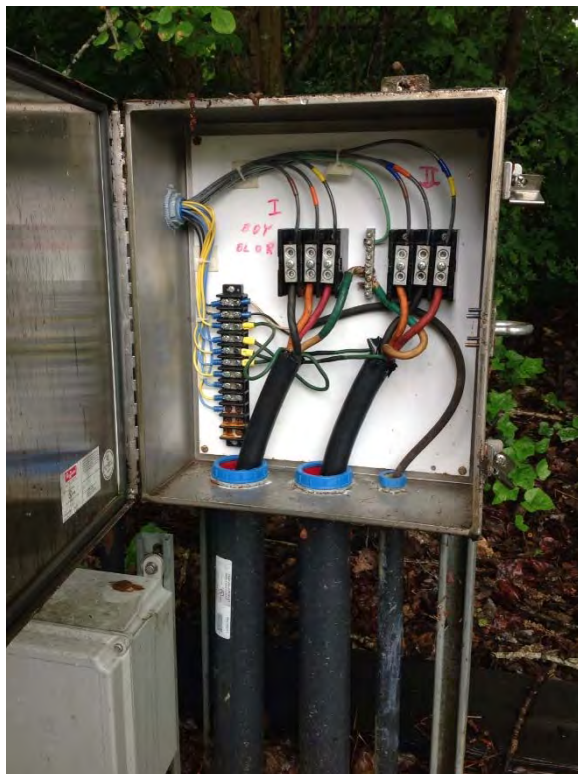
Submersible cable termination enclosure
