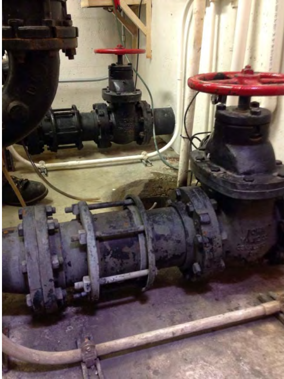
Gate valve isolation for suction piping
