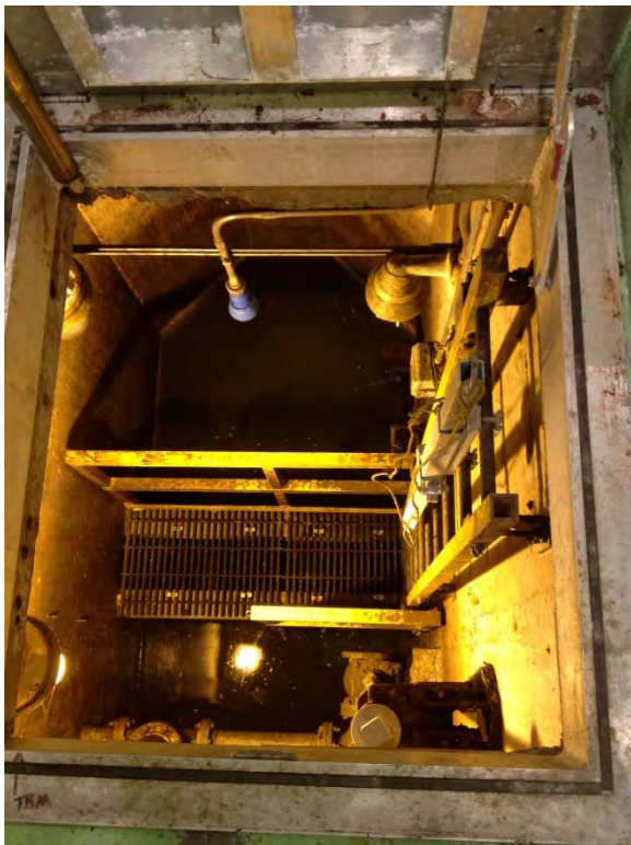
Interior of wet well appears to be in good condition
