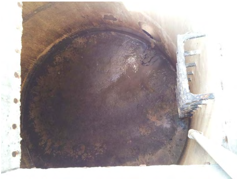
Interior of holding tank adjacent to wet well
