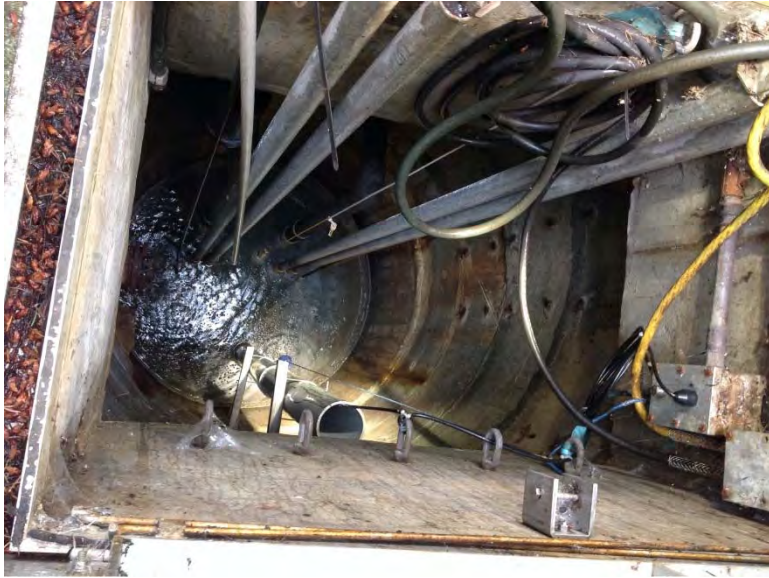
Submersible station, unable to observe pumps
