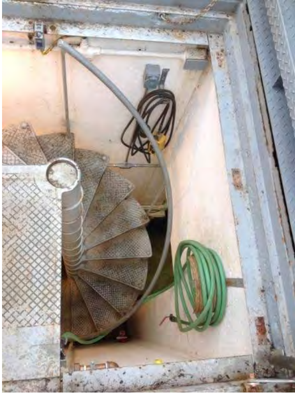
Spiral staircase appears to be in good condition
