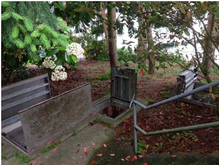
Six steps down to station from parking
