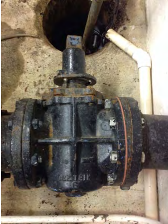
Suction plug valve – horizontal axis of rotation with seat to pump
