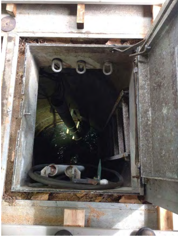
Submersible station, unable to observe pumps
