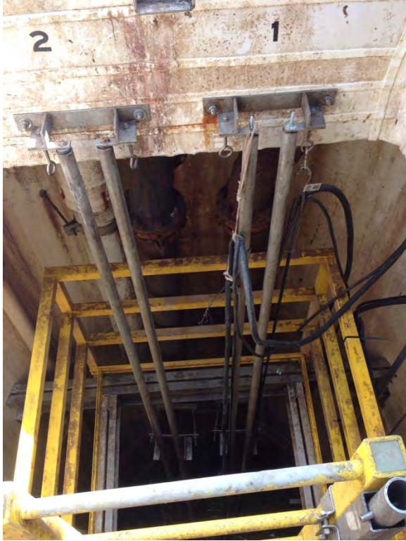
Submersible station, unable to observe pumps
