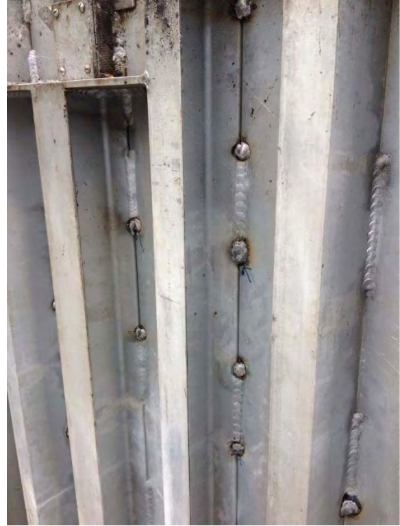
Wet well blower vault hatch, tacked up/re-hinged
