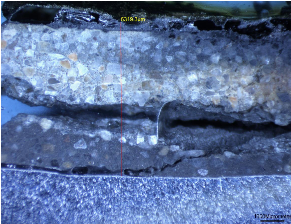
10x view of the cement layer on sample N-9 measured. There was no corrosion attack in the base metal.
