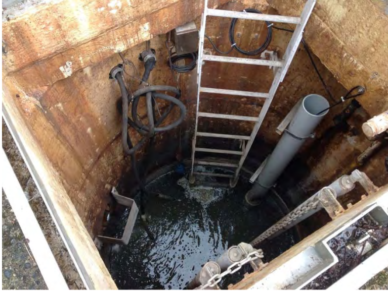
Submersible station, unable to observe pumps
