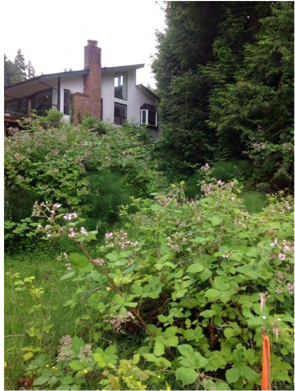
Generator receptacle located in homeowner's backyard in brambles
