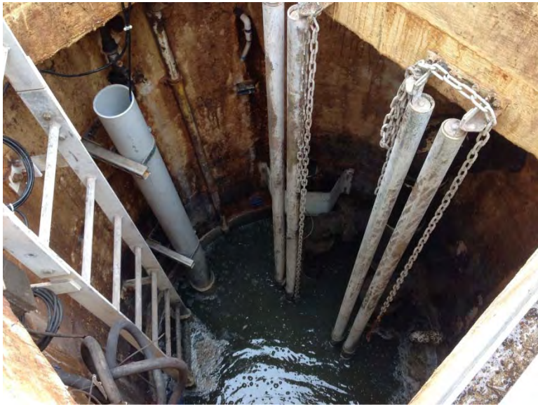
Alternate view of interior of wet well
