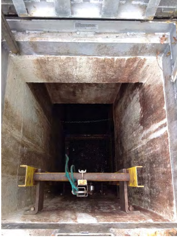
Interior of wet well
