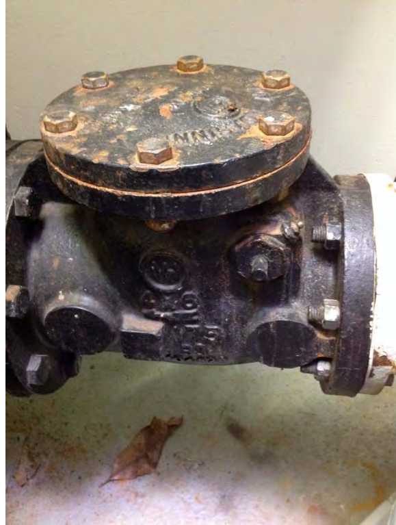
Swing check valve with outside weight and lever 4" x 6"
