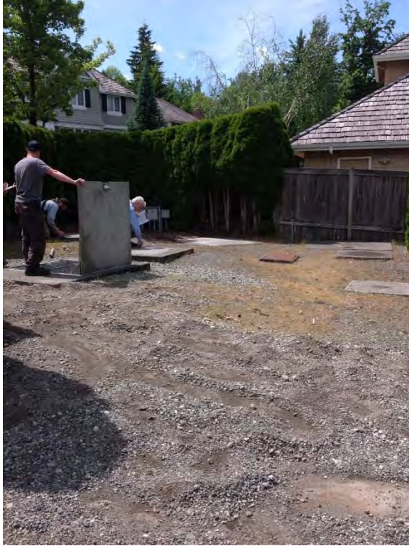
Hatches several inches above grade – potential tripping hazard
