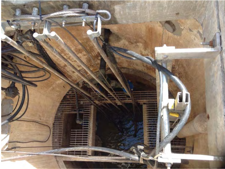
Submersible station, unable to observe pumps
