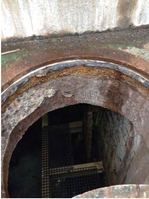
Interior of wet well, some exposed aggregate
