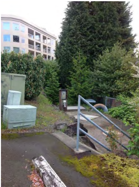
General site, stairs leading down to station – station is lower than adjacent parking
