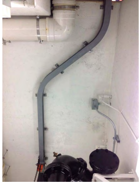
Ceiling of dry pit, rail with no equipment access hatch
