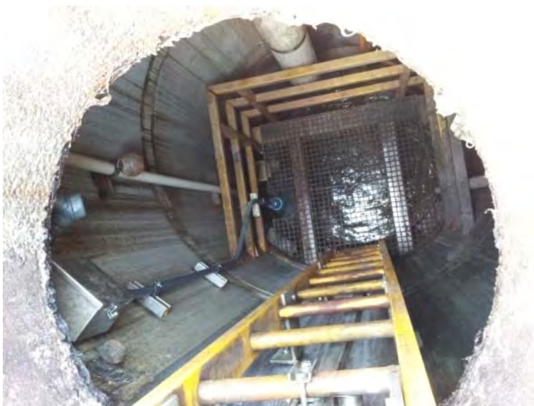
Interior of wet well
