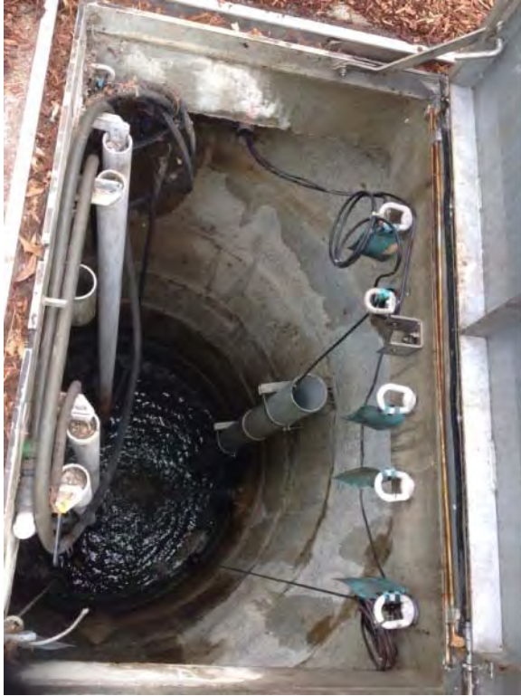
Submersible station, unable to observe pumps
