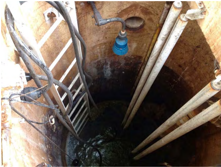
Interior of wet well appears to be in good condition
