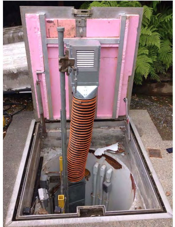
Fall protection available but you need to step over opening before latching on
