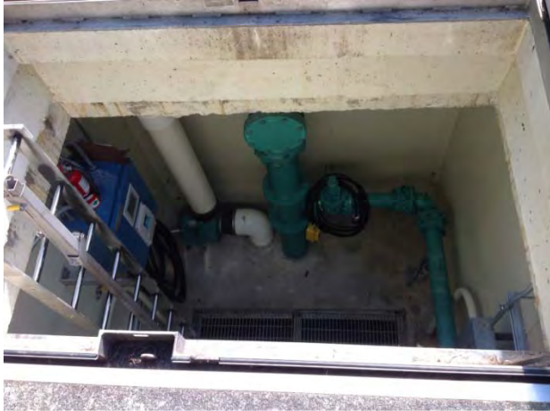
Interior of first floor of dry pit
