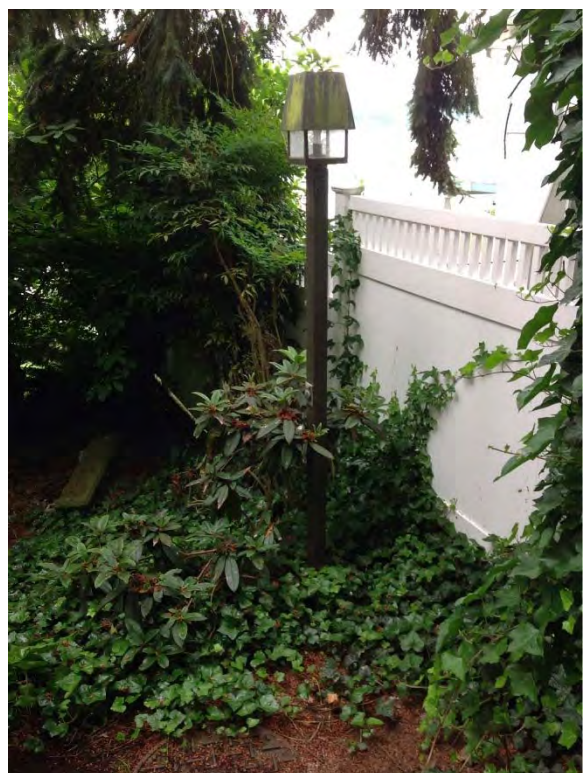
Site lighting adjacent to station
