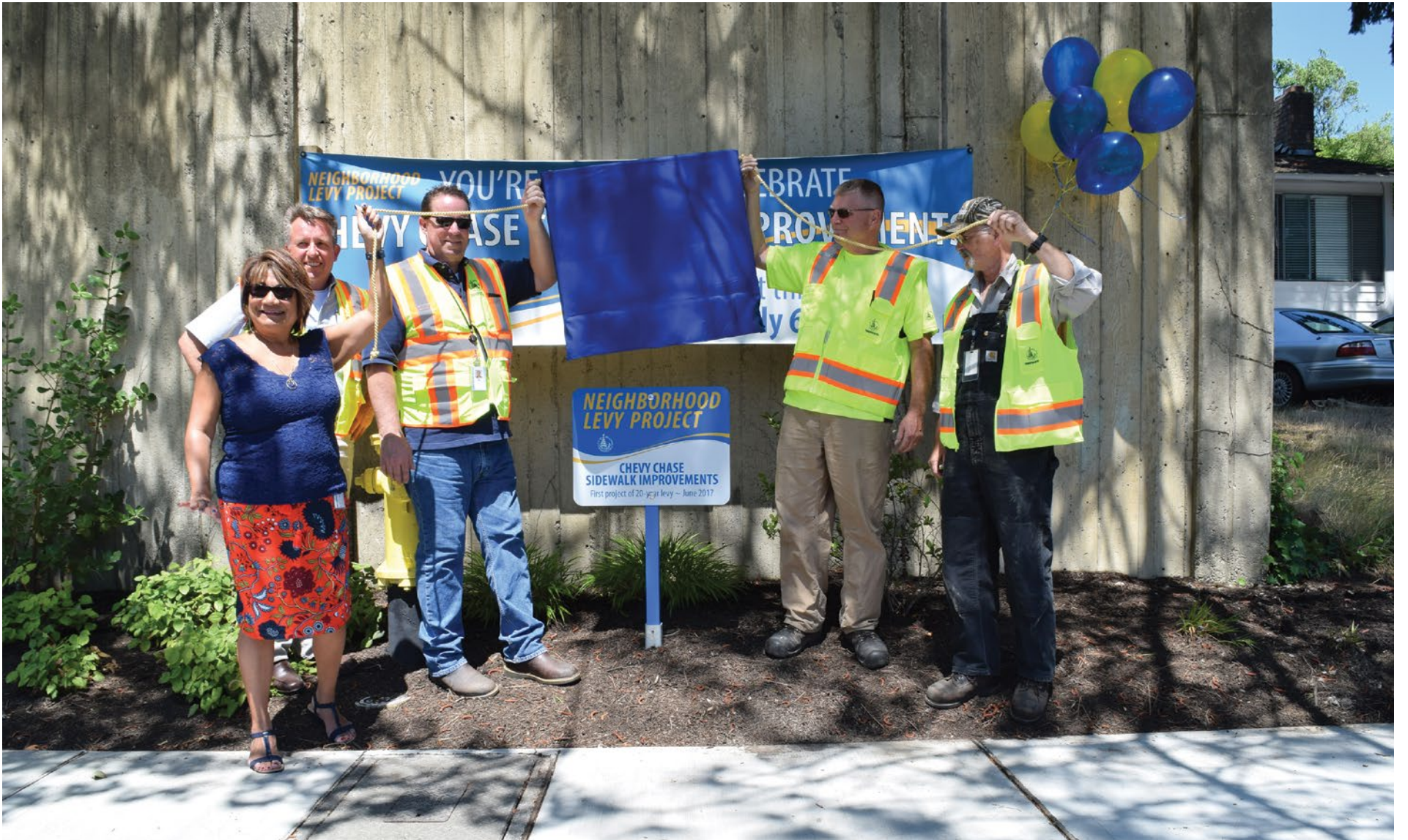
In June 2017, the first levy project kicked off, with 360 sidewalk panels repaired in the Crossroads neighborhood.
