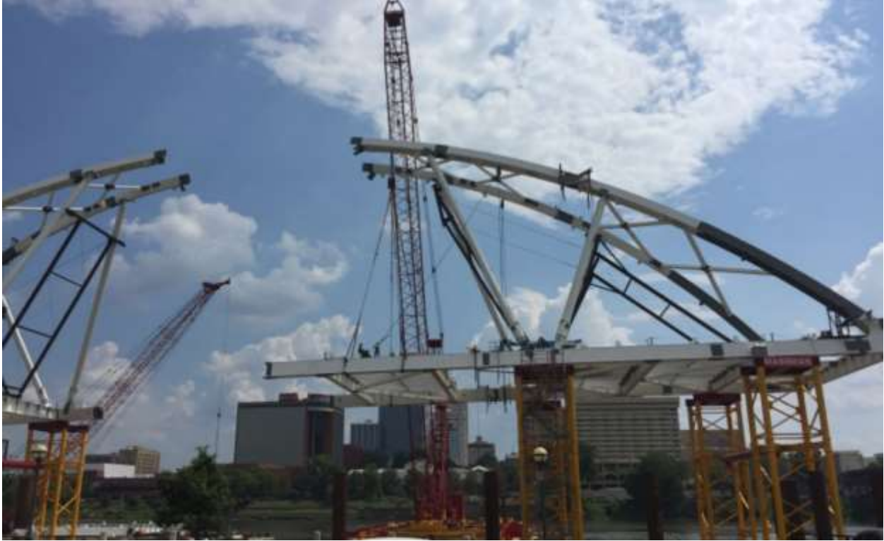
Figure 67: Construction of the Broadway Bridge in Arkansas. Segments of network-tied-arch supported by temporary support towers and temporary bracing (photo credit to Genesis Structures).
