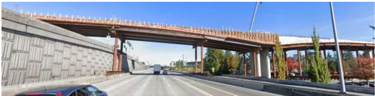
Figure 65: Falsework of Sound Transit's guideway structure on I-405 northbound traffic, looking north (photo credit to Google Map, Oct 2018).
